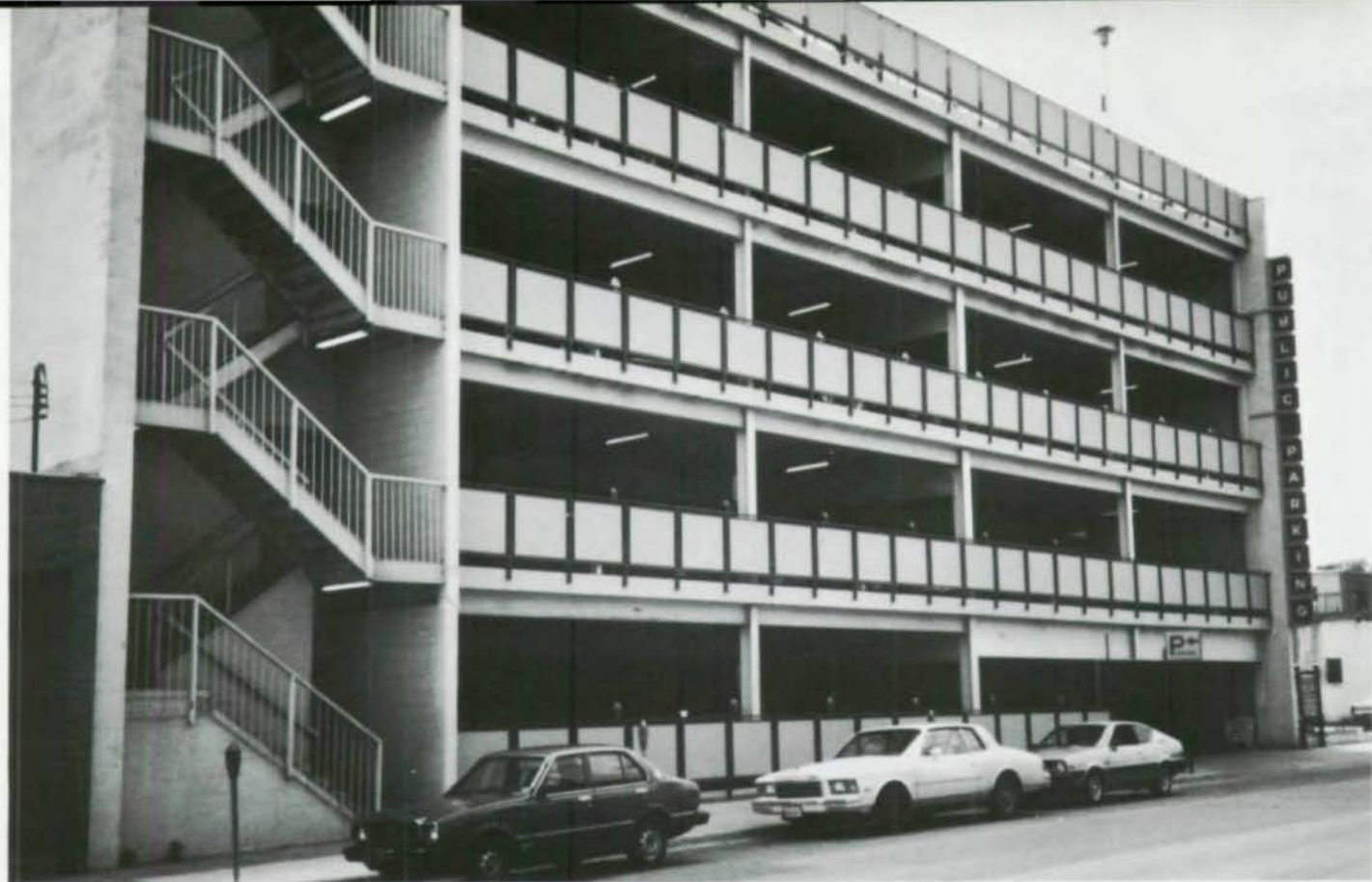
Security problems lessen when exterior open stairwells are designed into parking deck.
