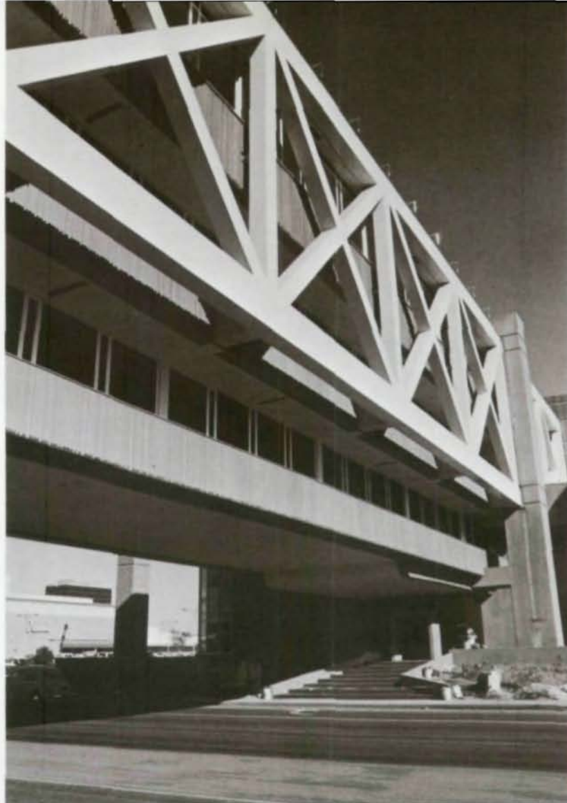
Pedestrian bridge was challenge. Fully enclosed, it joins three areas of hospital (above). Photo (l., below) indicates scale of 3-level bridge. Erectors (l.) hoist huge primary chord for pedestrian bridge.
