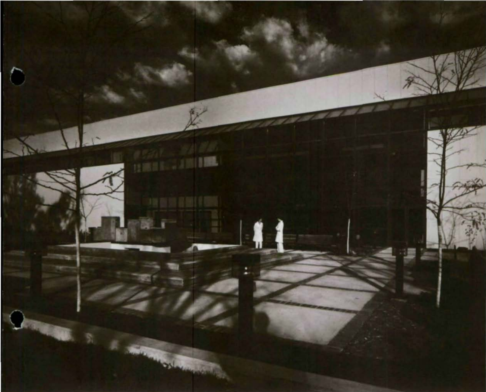
Phase II expansion of Billings Deaconess Hospital required unusual steel framing to meet special needs.
