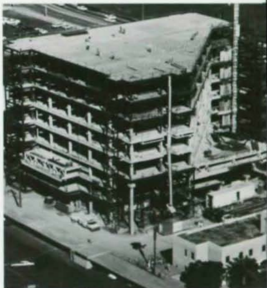
Congested conditions at hospital project required off-site staging of structural steel. Photo (bottom) shows interior of mechanical interstitial floor before equipment was placed.
