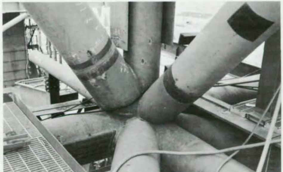
Service structure demonstrates huge amounts of steel used to withstand tremendous shock and heat of launch.
