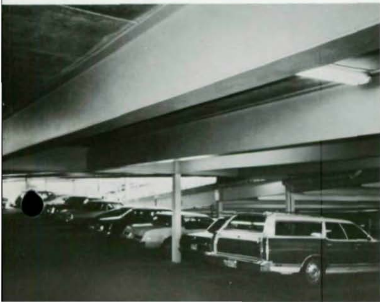
Steel framing painted in light colors (l.) saves on electrical energy costs. Steel on parking deck (r.) never received final field coat. Shop coat paint still in good condition after 13 years.
