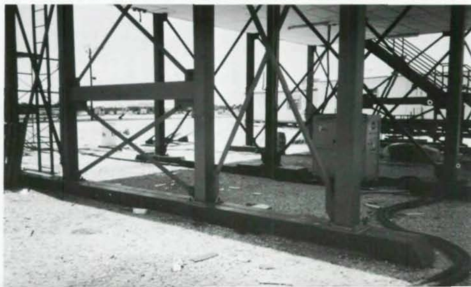
Tubular steel frame and tube feet provided fast-track solution to building quickly needed facility.
