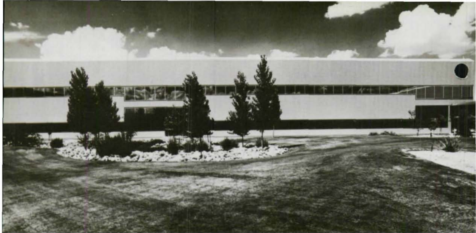
Horizontal ribbons of solar gray glass mirror desert sky in Tucson's new IBM General Products complex. Architects used modular approach in design of 1.7-million sq. ft in 18 buildings (below).
