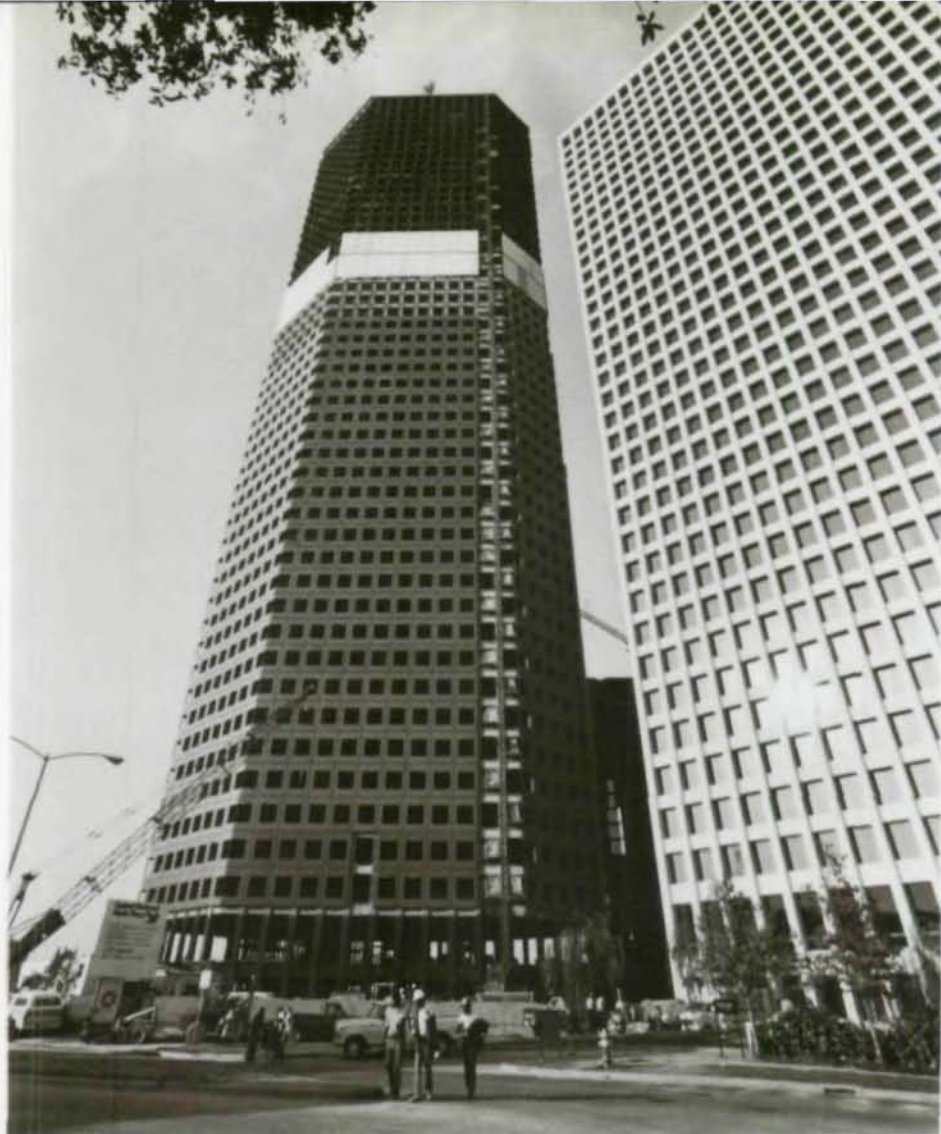
Under construction, steel-framed Capital Bank Plaza lends air of spectacular to Houston skyline.
