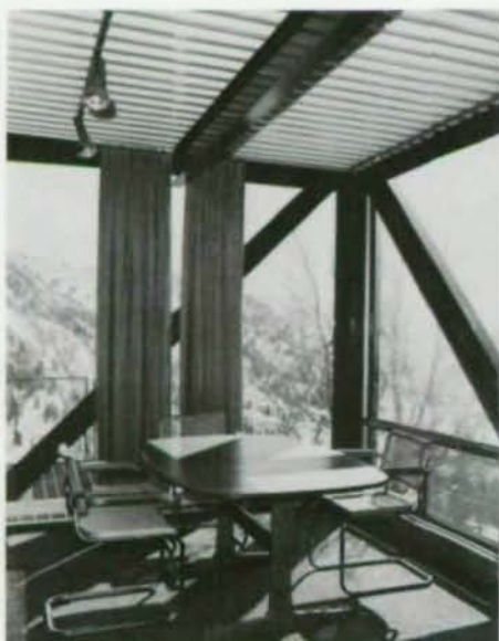
Tough describes terrain in retreat home of ski lodge manager. Shop-fabricated components eased construction, provided necessarily heavy steel framing for snow/wind loads.
