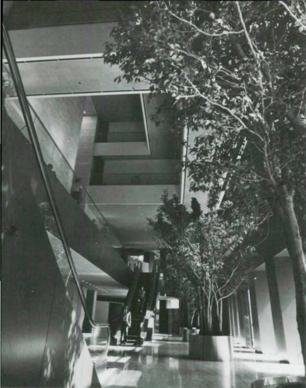
Magnificent four-story atrium, an "unplanned" event, was literally carved from steel frame already erected, to accommodate major bank tenant. Photo across page shows steel reframing in progress.
