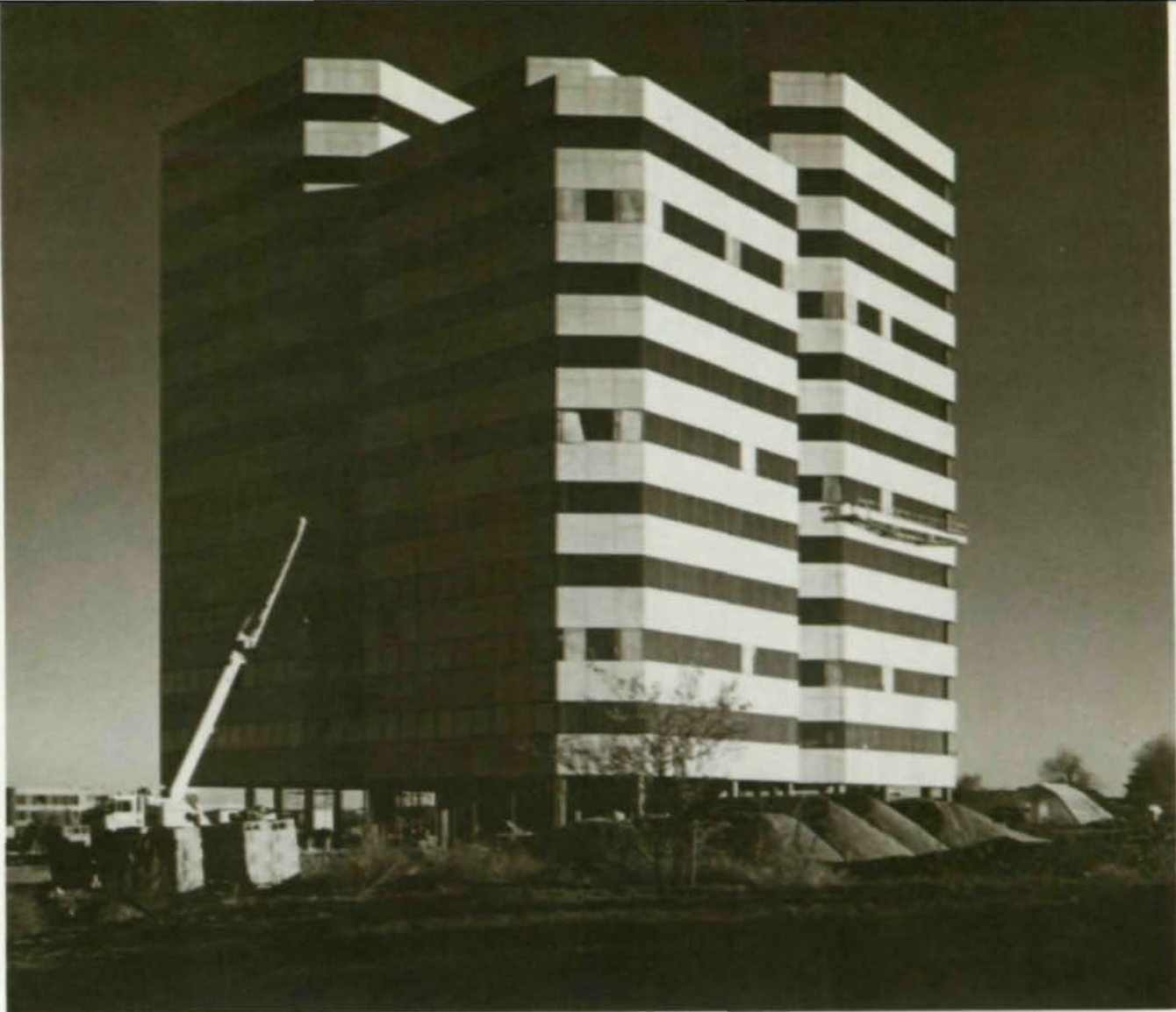
Terrace Tower 1, Denver, Colorado features new limestone cladding system over its steel frame.
