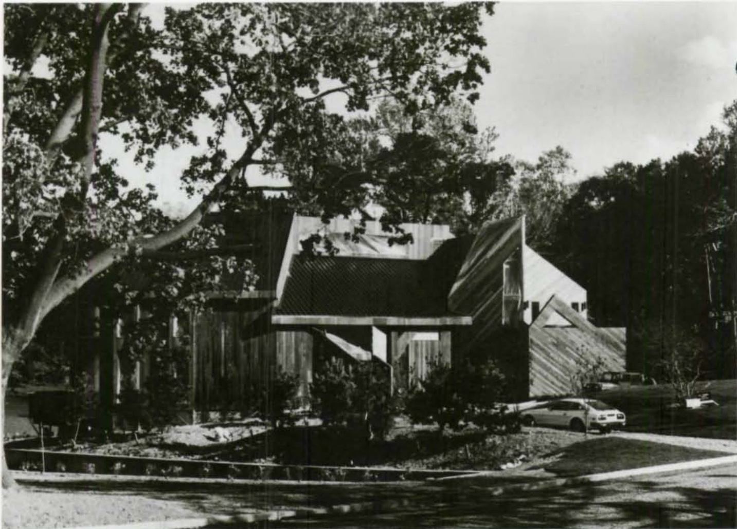
Owner who wanted view enjoys open planning of 5,400-sq. ft pond-side home. Steel framing provided maximum interior flexibility in floor planning.
