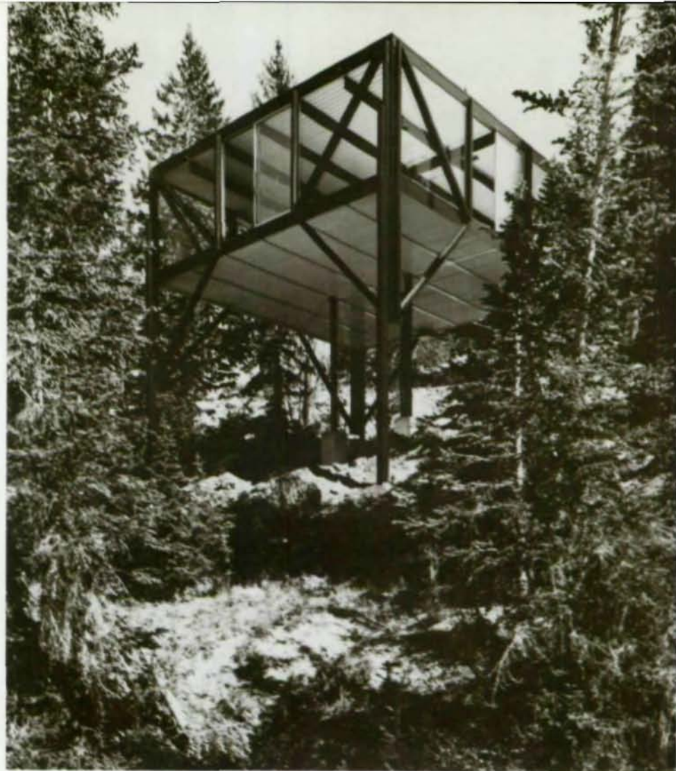
Remote mountain hideaway in picturesque setting features all-steel framing to minimize construction difficulties and provide partition flexibility.
