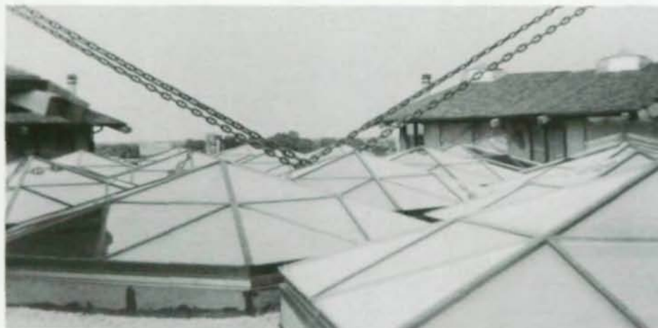
Dazzling skylight (far left) at luxurious Indian Lakes Resort (top left), Bloomingdale, Ill. features unusual structural steel framing details. Pyramid-shaped atrium (r.) provides intense natural lighting for guest rooms and dining areas below. Roof photos (l. and above) show hexagon grid details and massive ship chain supports.
