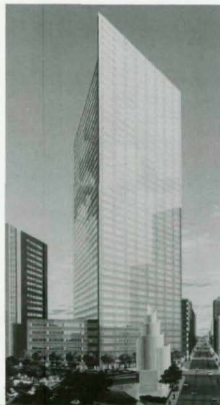
Figure 11—New Arco headquarters, Dallas
