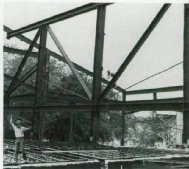
Giant 65-ft long x 15-ft high trusses go up to provide main roof support, enlarging central span and eliminating interior columns.
