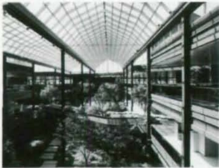
Deere & Co. headquarters, Moline, Ill. New Deere West addition (below) to 1964 structure was also built with weathering steel. Walkway/atrium ties two structures together.
