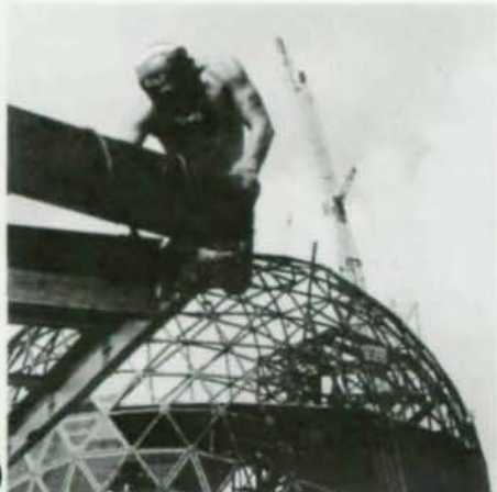
EPCOT Center, $1-billion Disney World addition (top), Orlando, Fla., fast approaches completion for Oct. 1 opening date. Eight million guests are expected annually. Steel-framed "spider"-leg platform (l.) is base for Space Earth, theme structure. Giant legs drop into place (c.). Photo (r.) shows structural details of unique sphere.
