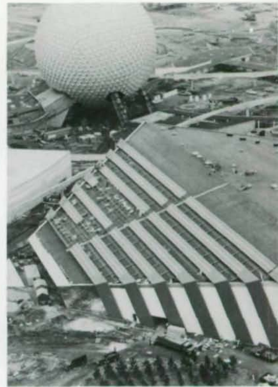
Exxon's Universe of Energy tells story of energy needs and alternate solutions for future. Roof has 80,000 photovoltaic cells to provide power.
