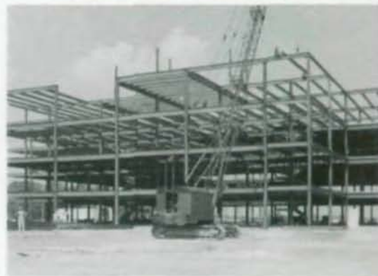
Structural steel frame made possible work around inclement weather and other delays.
