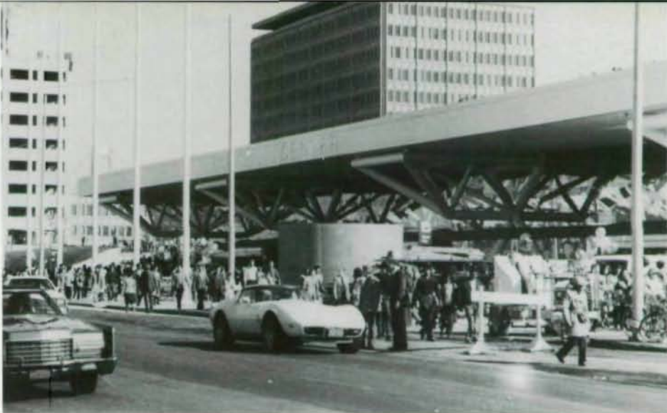
San Francisco's new Moscone Convention Center. Open street level lobby/atrium features four giant steel trusses that support roof (above & below).
