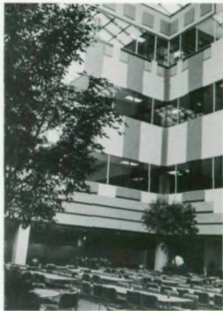
Handsome atriums, one in each side of building, house library and dining areas.
