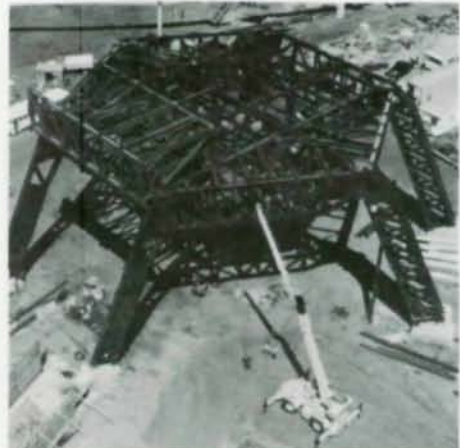
EPCOT Center, $1-billion Disney World addition (top), Orlando, Fla., fast approaches completion for Oct. 1 opening date. Eight million guests are expected annually. Steel-framed "spider"-leg platform (l.) is base for Space Earth, theme structure. Giant legs drop into place (c.). Photo (r.) shows structural details of unique sphere.
