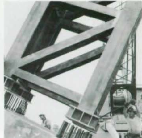
EPCOT Center, $1-billion Disney World addition (top), Orlando, Fla., fast approaches completion for Oct. 1 opening date. Eight million guests are expected annually. Steel-framed "spider"-leg platform (l.) is base for Space Earth, theme structure. Giant legs drop into place (c.). Photo (r.) shows structural details of unique sphere.
