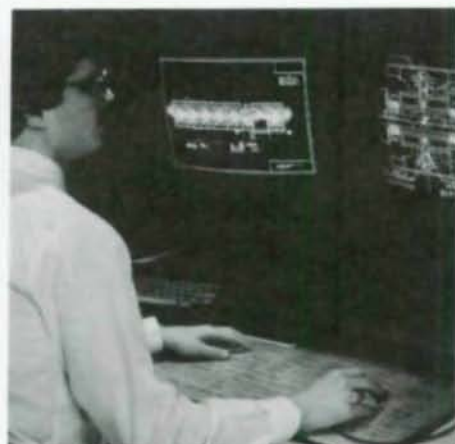
Major architectural/engineering firm pioneers use of computer graphics in design. In background (l.), main frame computers, disk storage units and plotter (r.). Digitizers (above) speed routine drafting work.
