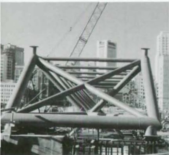
Longitudinal seismic forces are transferred to huge trusses by double-angle K-bracing. Construction photo (above) gives idea of size.
