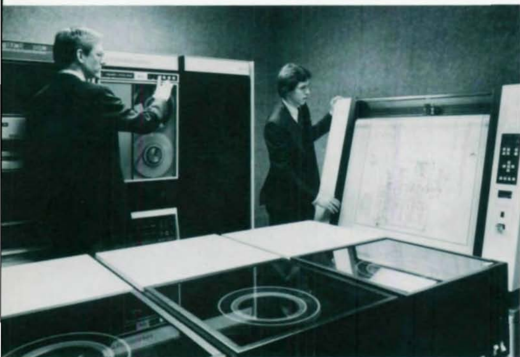
Major architectural/engineering firm pioneers use of computer graphics in design. In background (l.), main frame computers, disk storage units and plotter (r.). Digitizers (above) speed routine drafting work.
