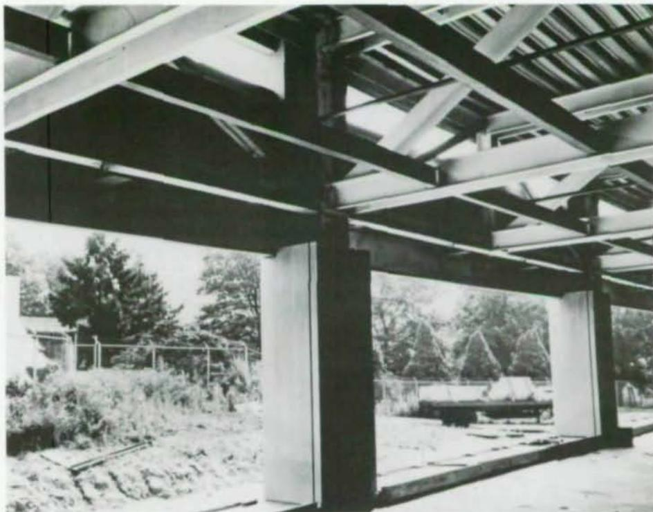
Modified Warren trusses (L) support interstitial spaces, permit column-free patient areas and full access for service lines. Bottom of steel flooring (above) is visible above interstitial area framed by network of steel girders.
