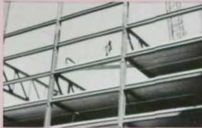
Closeups detail K-bracing (l.) and spandrel end plate design (below).
