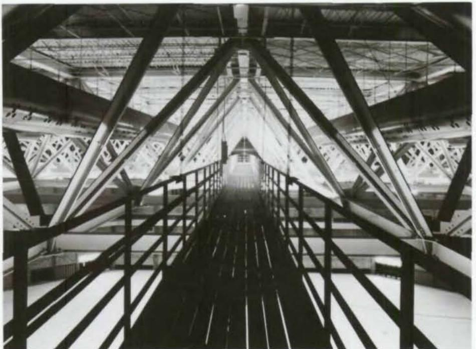
*Truss system provides ample room for large duct system to feed through it, reduces building cubage and gives maximum head-room for athletic events.*
