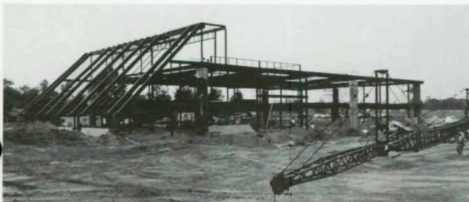
*Sloping, energy-efficient glass facade lends air of distinction to new Hillier Group headquarters building (far l.) in Princeton, N.J. North-facing windows permit indoor daylighting. Steel frame (l.) was architect's choice for its economy and speed of erection.*
