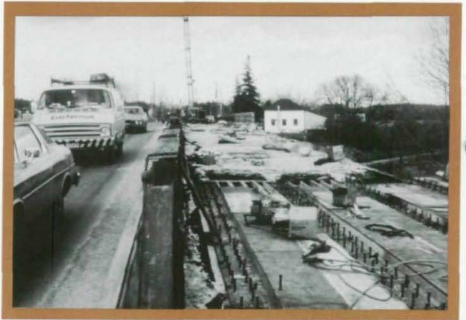
*Deteriorated deck (top) was reconstructed (bolt.) using half of bridge width to maintain traffic.*
