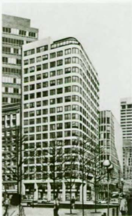
The 18-story 155 Federal Street Building had to "match" existing 10 High Street in historic area. Unusual steel framing details did job while tenants remained in building.
