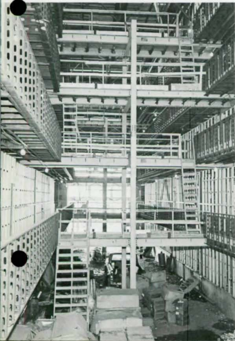
Historic Charlestown Navy Yard building (l. pg.) were transformed into handsome apartments below. Steel framing (l.) permitted extensive structural renovations required.
