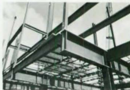
Multi-story rigid frame provided low cost and ease of construction for luxury condos.
