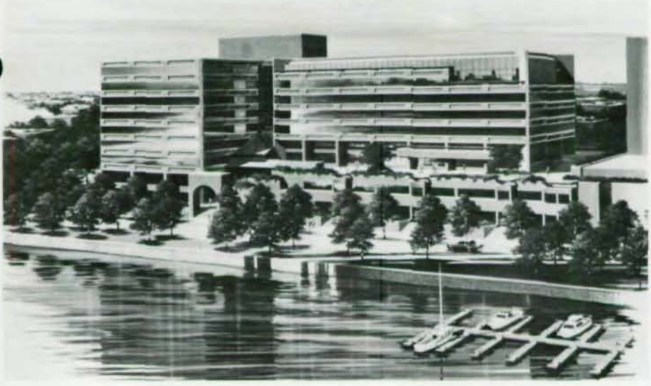
Riverside Place, Cambridge, office building
