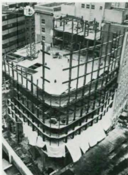
Original site condition (top) exposes area of 30-ft sq. light well which became service core. Bird's eye view (bottom photo) midway through steel erection shows moment frame trees to 12th floor, core framing in background.
