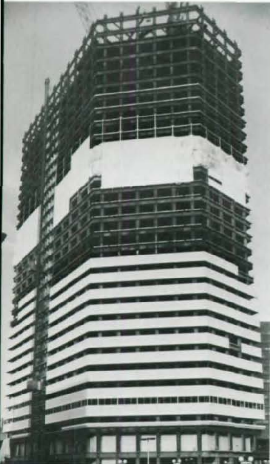
Steel-framed Dewey Square (l.) nears top out. Above, isometric shows perimeter steel framing.
