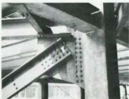
Typical connections at reentrant corners (top); typical connection at bracing detail (bottom photo).
