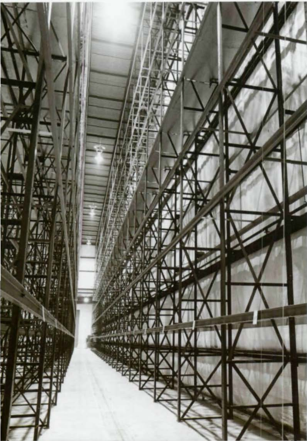
Typical end wall (l.) of Fay's Drug Co. warehouse, Liverpool, N.Y. Photo (r.) shows typical 4-in. structural channels, beams and columns. Photos by Klineberg.
