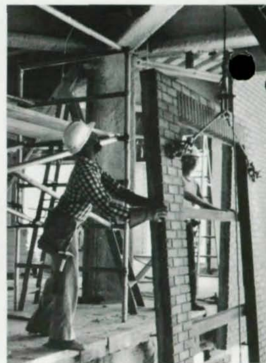
Precast panel installed under floors spanning across walkway.
