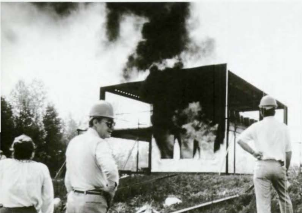
Full-scale burnout test at NBS simulates high-rise office fire. Early results confirm computer's ability to predict steel frame performance in a fire. U.S. Steel photo.
