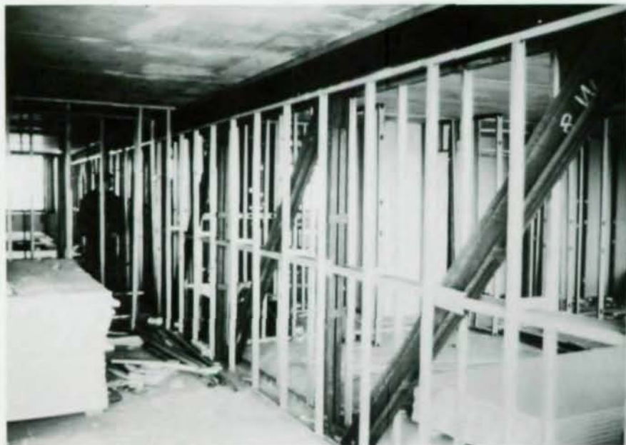
Mockup for truss protection within a hotel wall erected for UL fire test.
