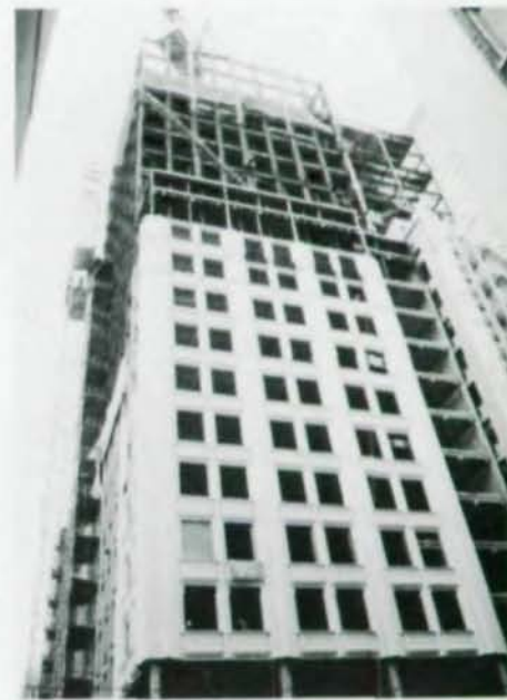
Photo 6 (l.). Inside face of prefab terra cotta panel shows backup system used to attach panels to structural steel frame. In Photo 7 (r.), one-story panels are attached to steel frame. Prefab technique was key to matching old and new structures.
