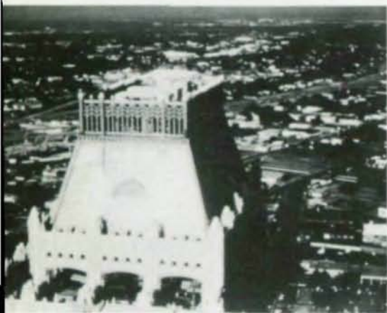
Fig. 1. Copper-clad grillwork encloses mechanicals, tops off truncated pyramid walls.
