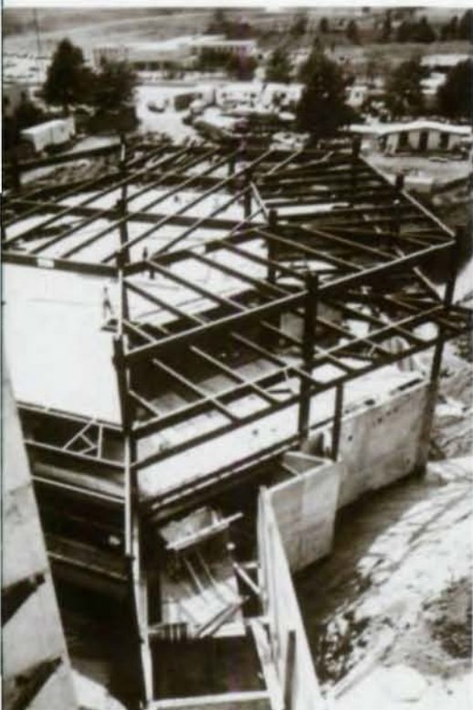
Fig. 1. St. Francis Hospital. Photo shows girder layout for hexagon-shaped 11-story moment-resisting frame.
