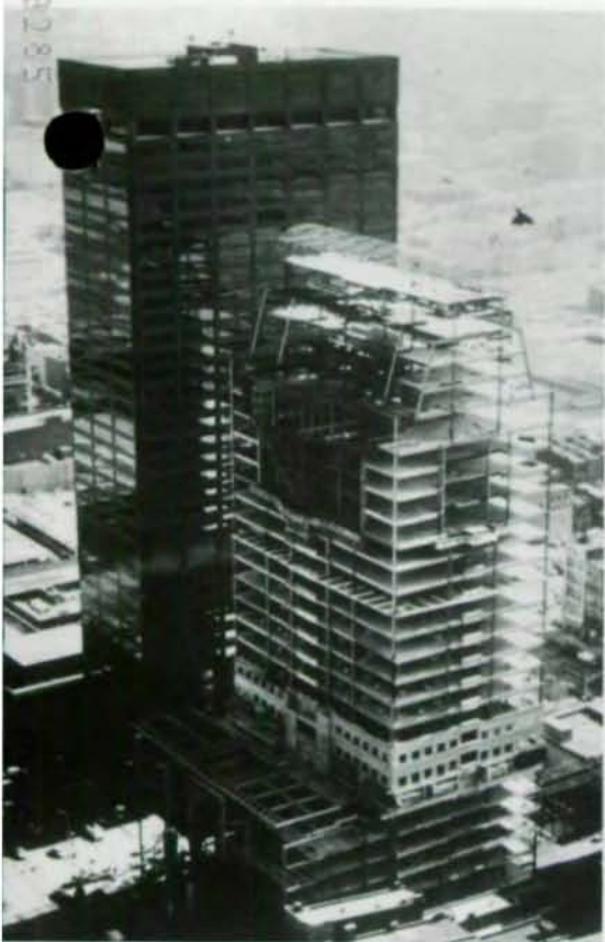
Fig. 5. Humana Corp. headquarters. Structurally complex building required design of nine separate frames.
