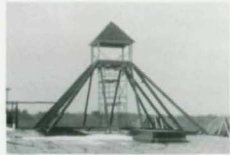
Four large cupolas (r.), designed in steel for ease of construction, grace entrance canopy. Steel framing details diagramed below.
