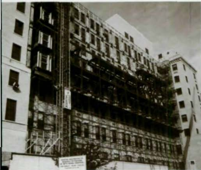
Fig. 1. Overview of new structure (above) with steel framing partially erected. Support collars at existing columns can be seen at upper floors. Fig. 4. Overview of framed brackets (above, r.) and tube column on left which provides interdependency between each bracket. Fig. 5. Support assembly with partial framing (r.) shows bolting of faceplate into existing column.
