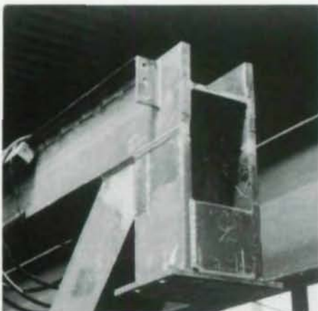
Fig. 6. Main roof trusses (above) were assembled on trading floor deck and erected by two cranes.
