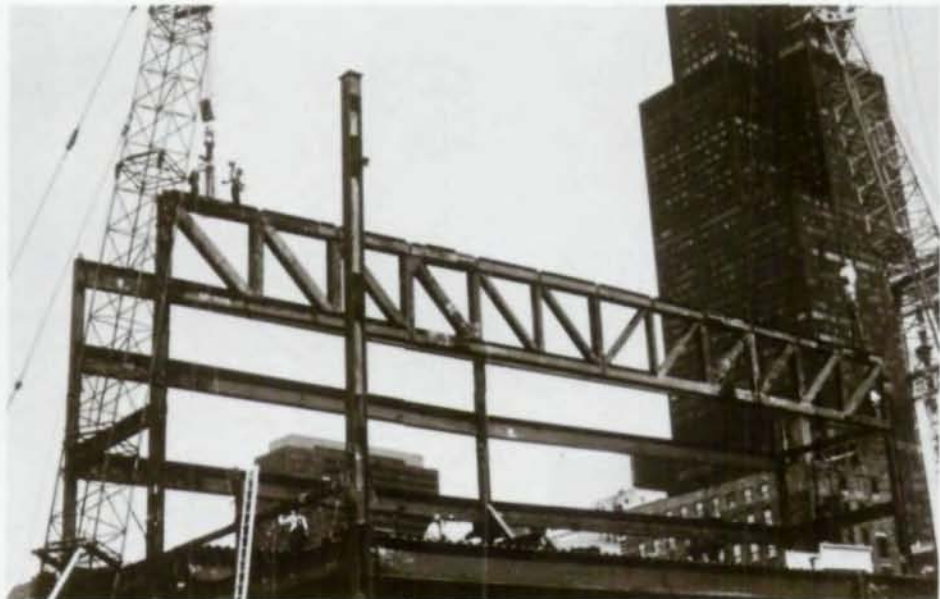
Fig. 6. Main roof trusses (above) were assembled on trading floor deck and erected by two cranes.
