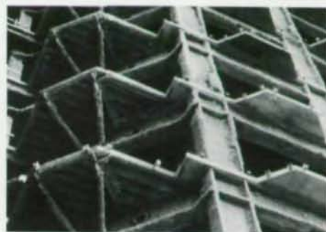
Fig. 3. Typical 45° corner spandrel condition and cantilevered floor slabs, creating bay window articulation.
