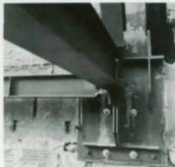
Fig. 1. Overview of new structure (above) with steel framing partially erected. Support collars at existing columns can be seen at upper floors. Fig. 4. Overview of framed brackets (above, r.) and tube column on left which provides interdependency between each bracket. Fig. 5. Support assembly with partial framing (r.) shows bolting of faceplate into existing column.
