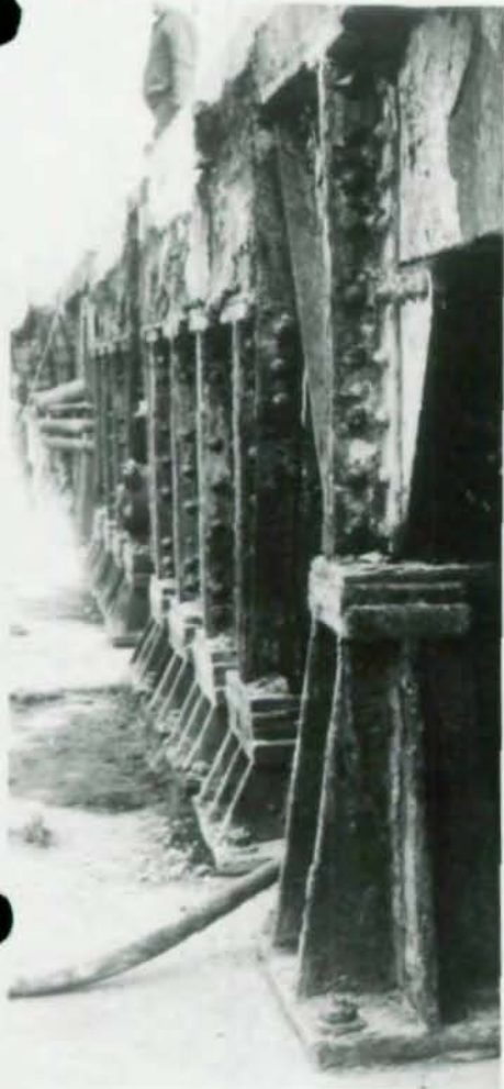
Fig. 5. View of girder bearings at north pier shows localized corrosion, areas that were cleaned and repainted.
