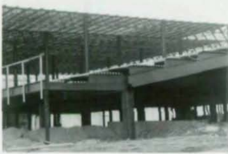
Stepped grandstand (l.) shows steel framing, with typical step detail (below, l.).
