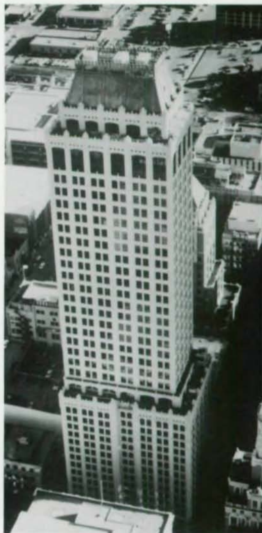
Fig. 2. Mid Continent Tower. HTB used SPACE IV structure analysis on 37-story steel framed-tower.
