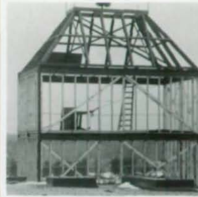
Photo booth framing is combination of steel and light steel wall studs. Detail on left.
