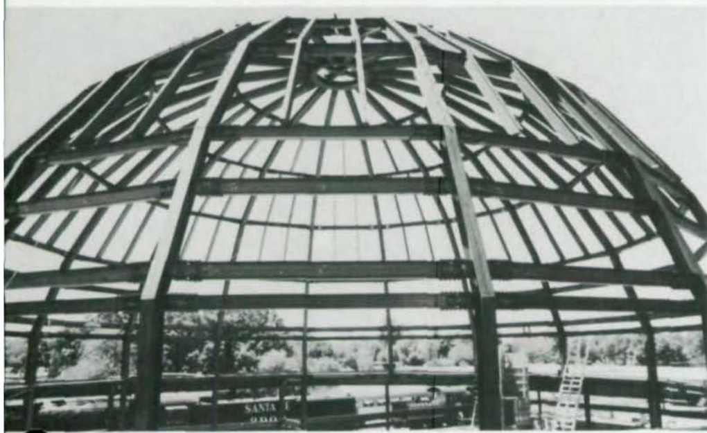
Intricate steel-framed dome is one of more popular and economical types.
