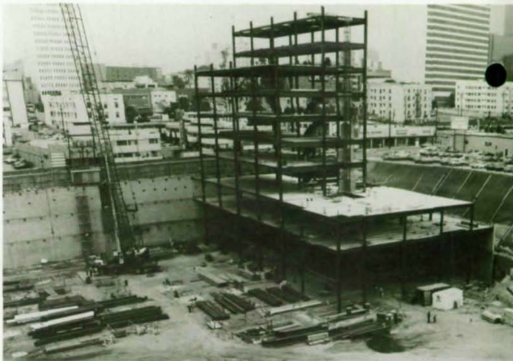
Steel-framed building was fast tracked to permit tie-back shoring and placement of basement walls during steel fabrication.
