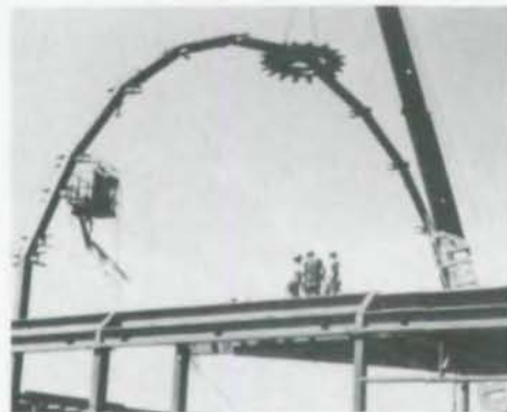
Interesting erection photos (above) show compression ring swinging into place.
