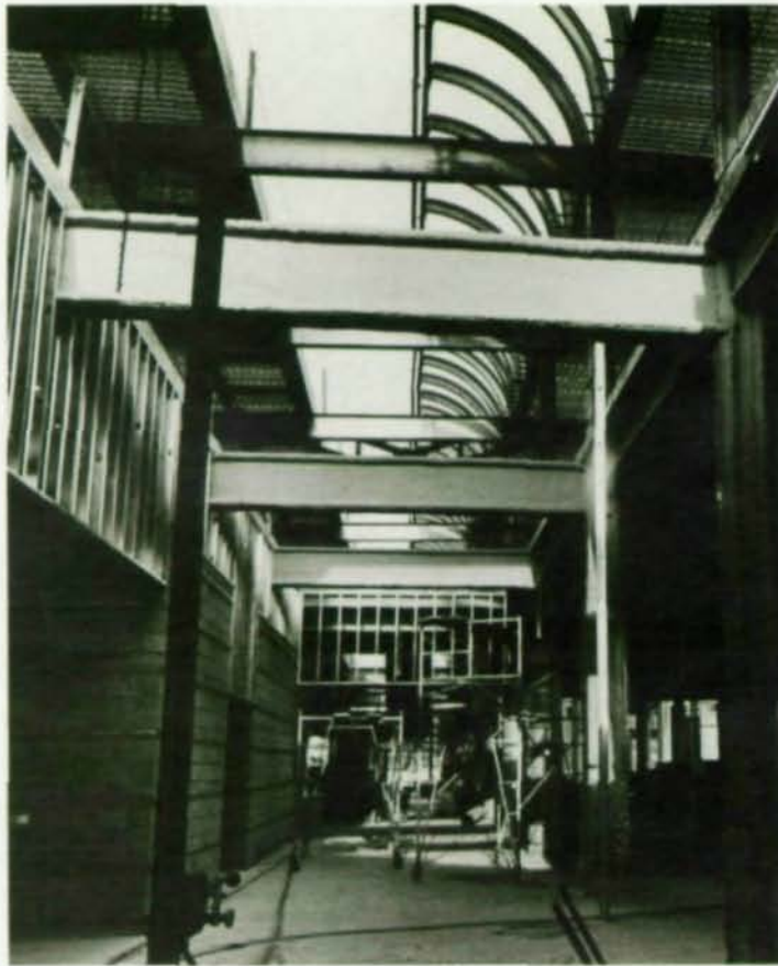
Steel-framed atrium zone joins addition to existing facility.
