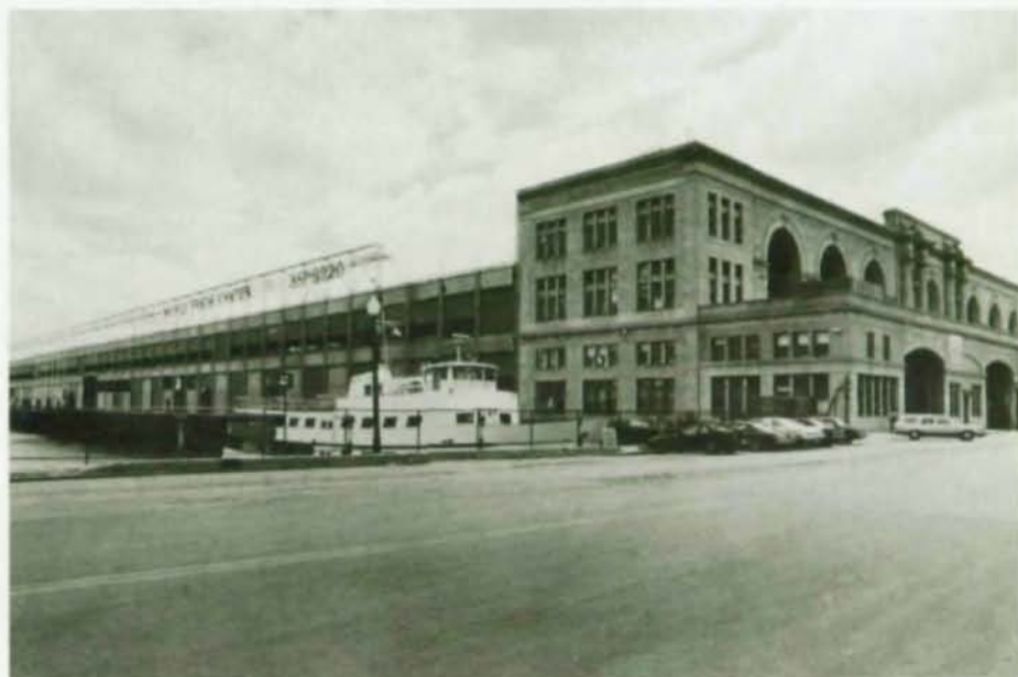
Boston's new World Trade Center (top) is remodeled Commonwealth Pier (bottom). Fast tracking was major consideration in exciting renovation project.
