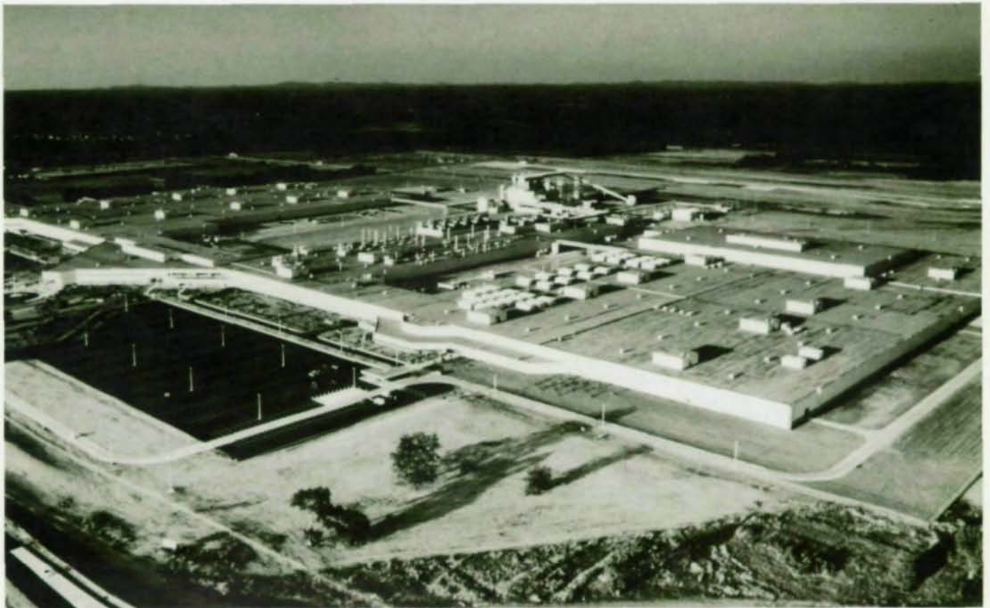
Aerial photo of finished car assembly plant displays mass of project.
