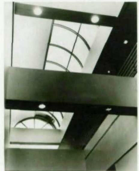
Interior photos highlight several uses of structural steel to accommodate skylights and overhang framing.
