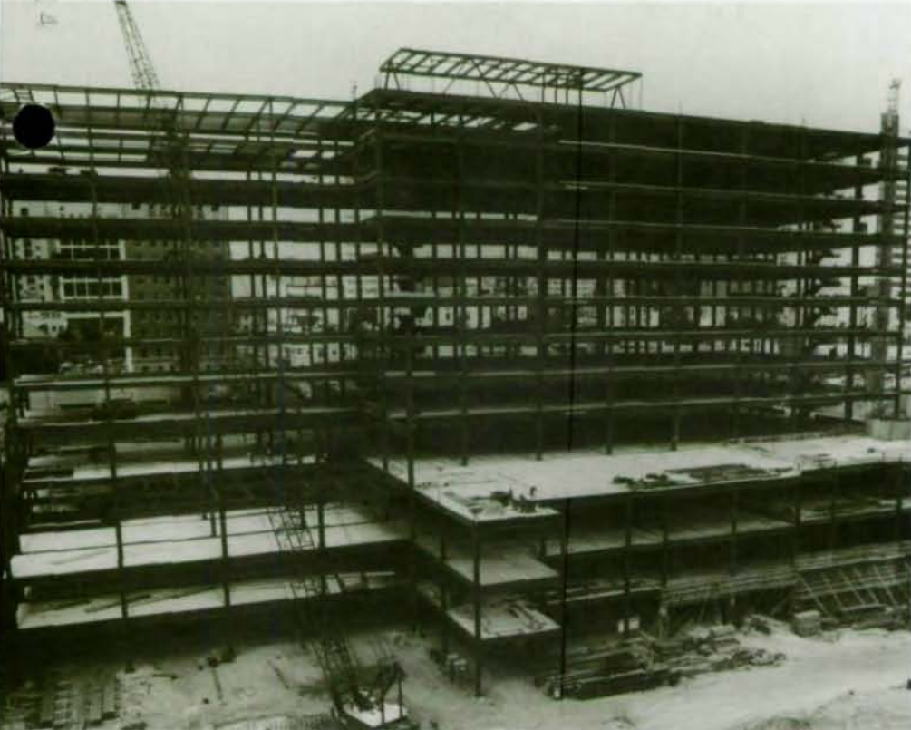
Structure is four interconnected modules designed to support a future 21-story building.
