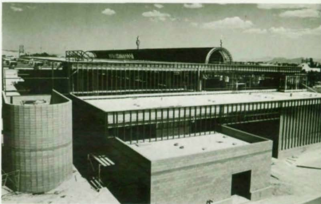
Structure was designed with moment-resisting frames. Horizontal X-braces provide continuous roof opening to frame skylights.
