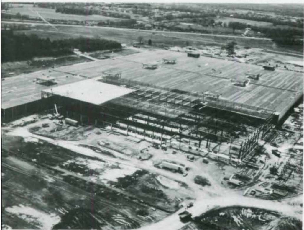
Nissan Motors building transformed 782 acres of pasture into state-of-art assembly plant. More than 14,000 tons of steel framing went into 2.8-million sq ft facility.
