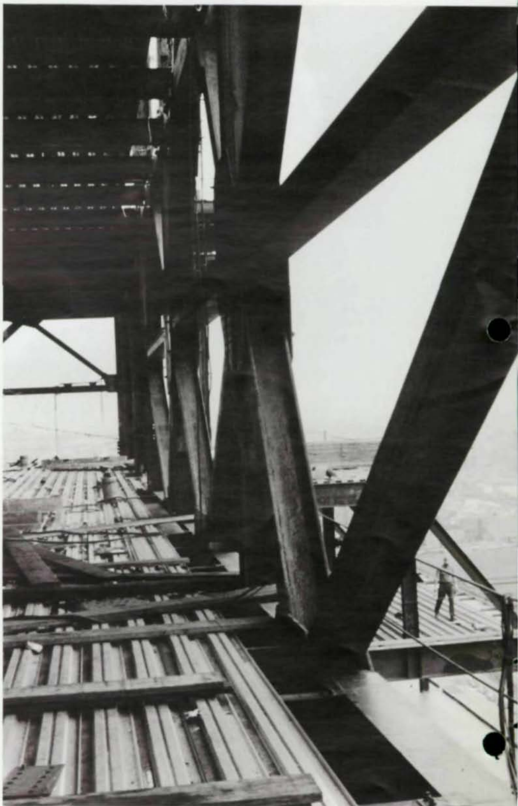
Wind bracing line at 17th floor in building's north face
