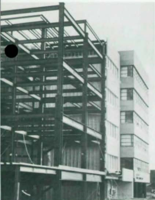
Steel-framed construction occurred without disrupting building use and regardless of weather conditions.
