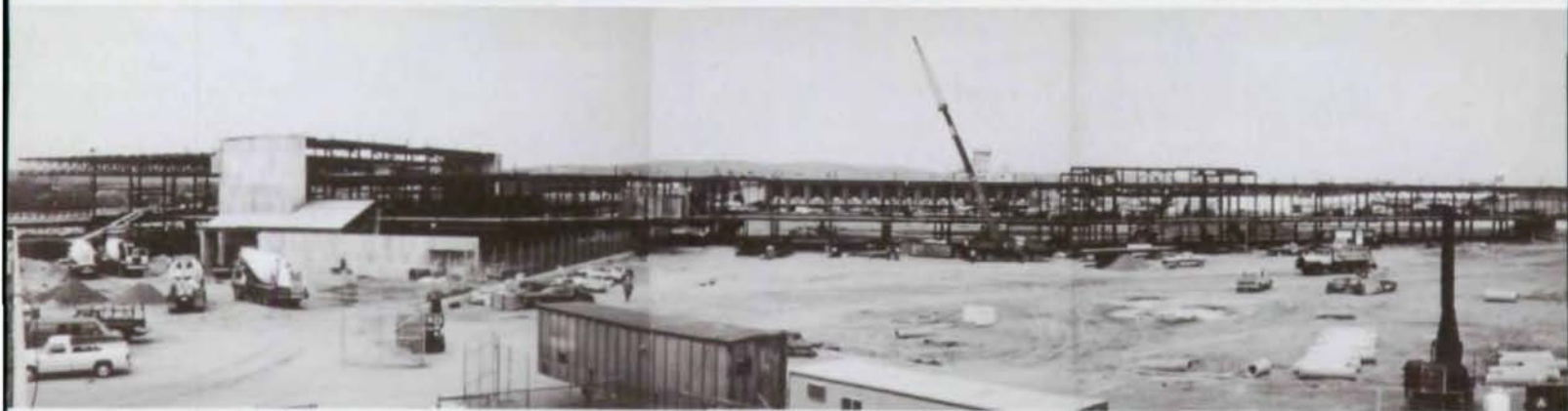
Composite photos of Bradley Airport show extensive addition to congested airport facilities. Steel framing accommodated design, sped construction.
