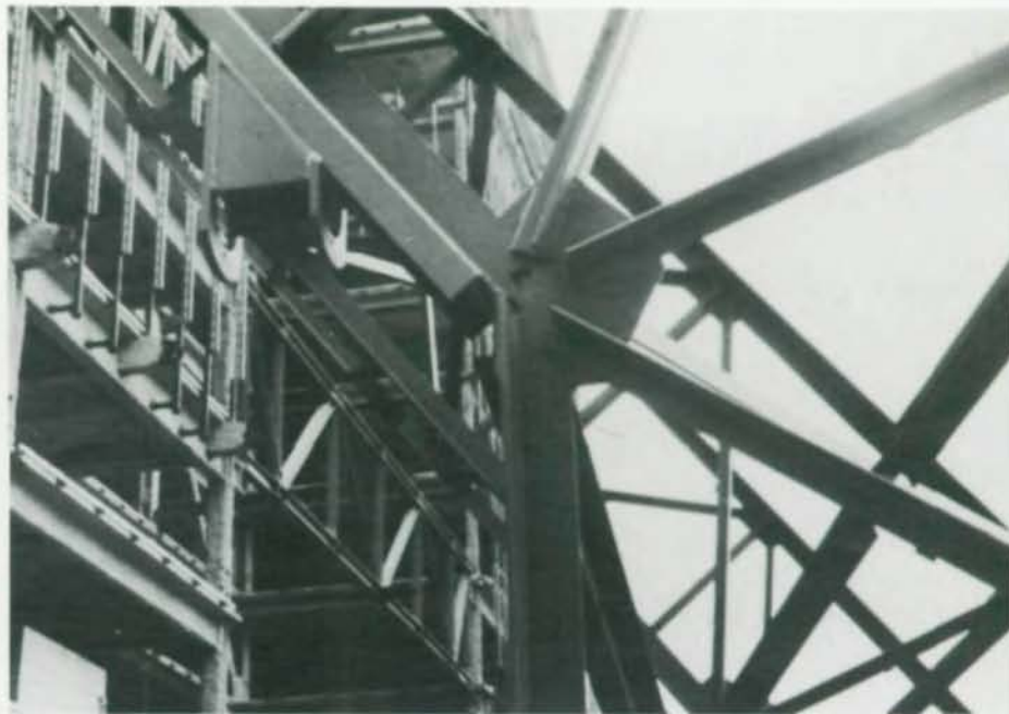
Angulated truss support and 13ft-5 in. deep truss supporting 90-ft wide indentation
