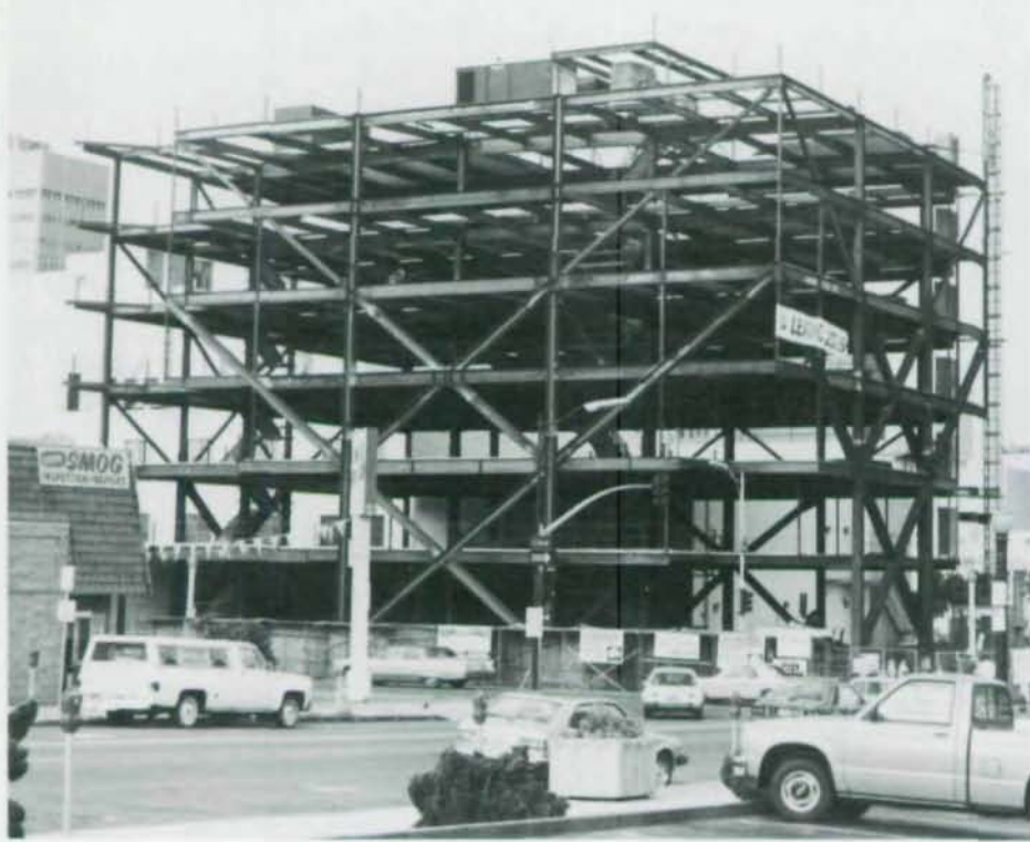
Site limitations on Ticor building were overcome by architect in using diagonal braces to increase floor areas and improve visual appearance (l.). During early construction, crane dropped equipment into hole to work.
