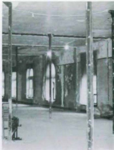
Steel trusses in 3rd floor (l.); and floor hangar supports (c.) over waiting room. Modification to existing trestle support (r.)
