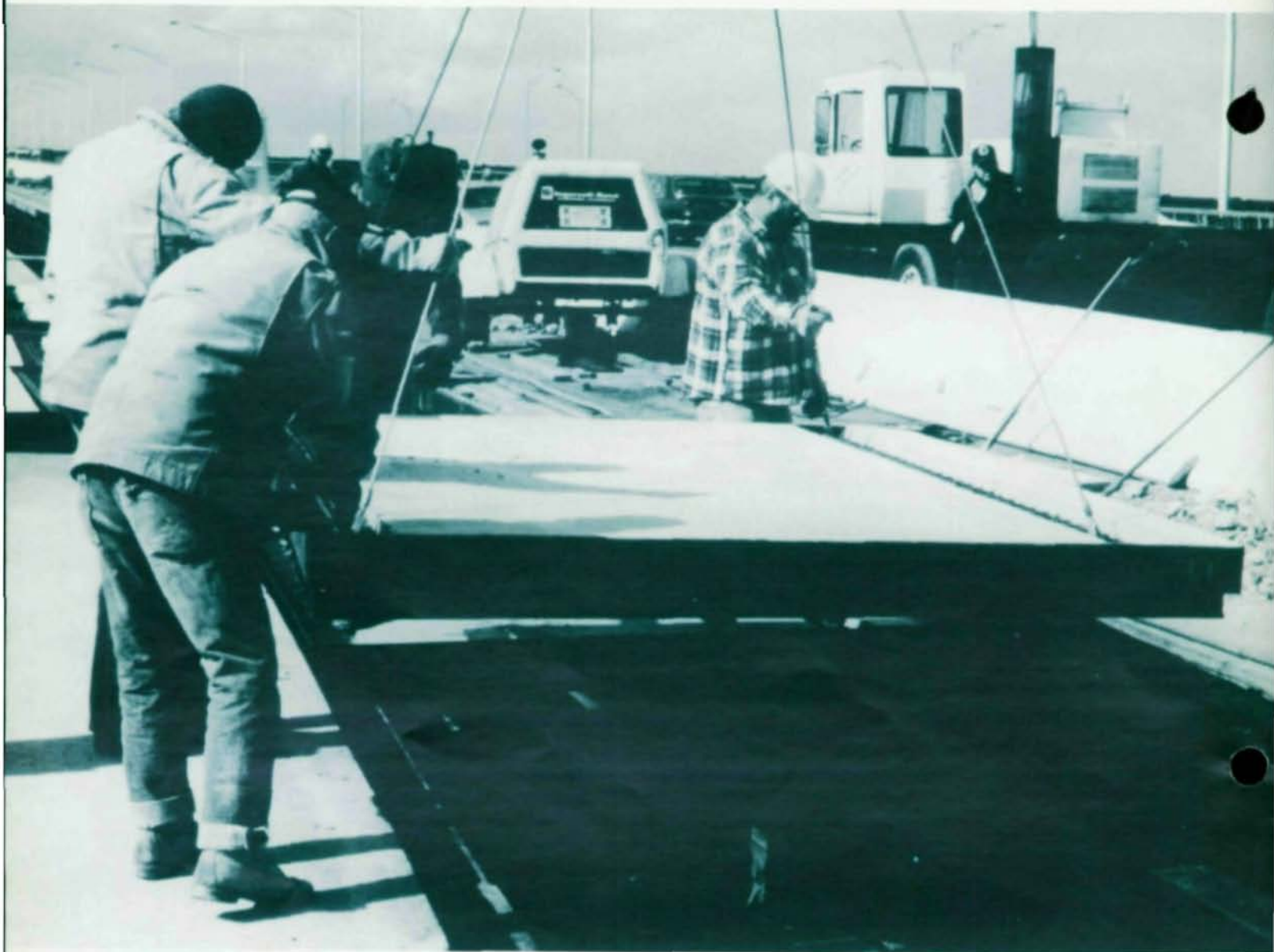
Exodermic deck panel is installed on Driscoll Bridge, one of 564 panels replaced.
