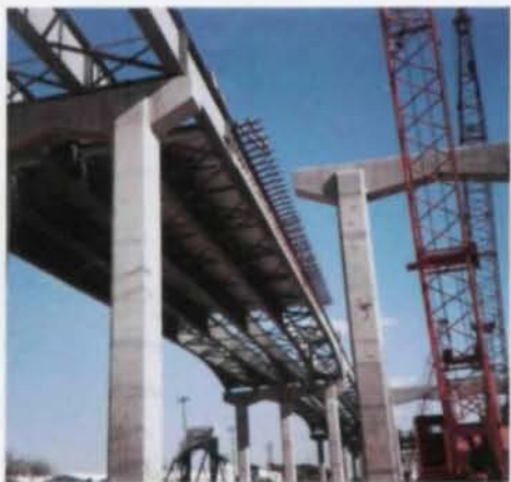
To reduce bridge construction costs on a 12-foot span, Bowman LSM deck forms have been used on the I-95 overpass in Broward County Florida, near Ft. Lauderdale.
