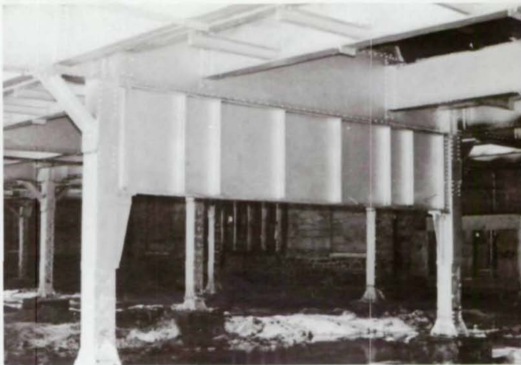
New plate girder supports trestle of remodeled depot.
