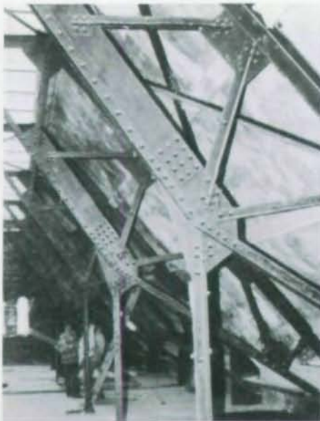
Steel trusses in 3rd floor (l.); and floor hangar supports (c.) over waiting room. Modification to existing trestle support (r.)
