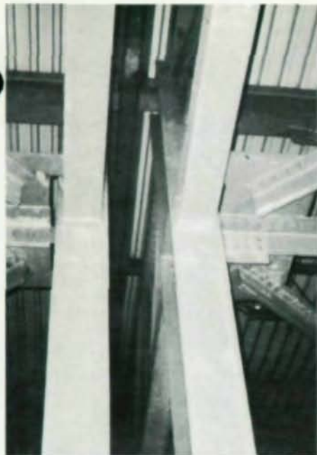
Connections under metal decking
