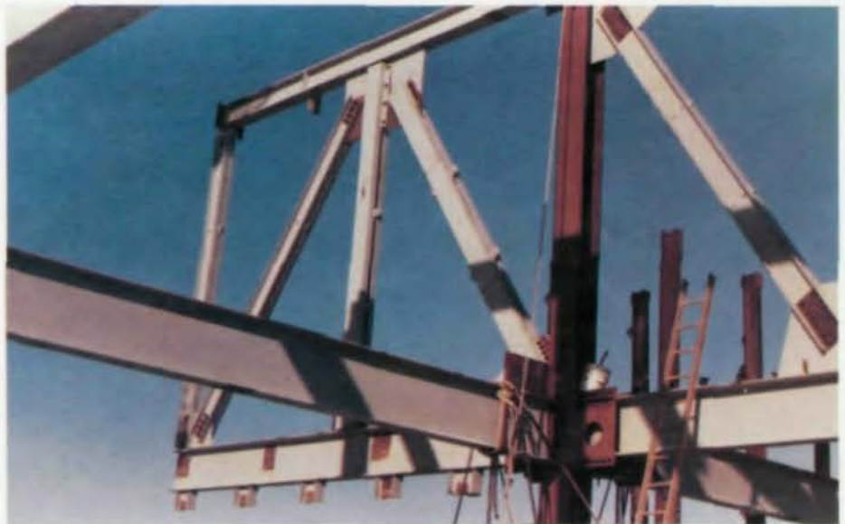
Trusses cantilever up to 26 ft at roof level to form distinctive architectural crown.
