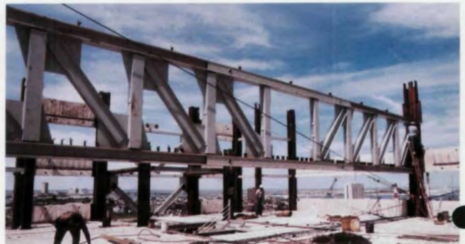
Typical truss is bolted. Note shop-applied channels on bottom chord, shear studs on top for critical shear force transfer between slabs and trusses.
