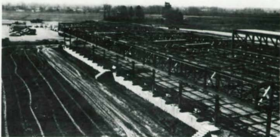
Line haul building during erection.
