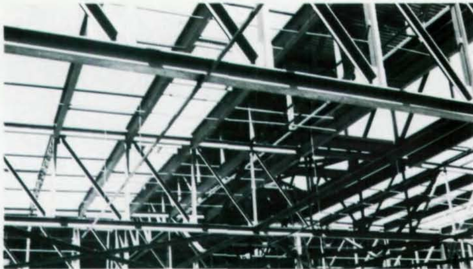
Extensive use of structural framing looking toward sort building
