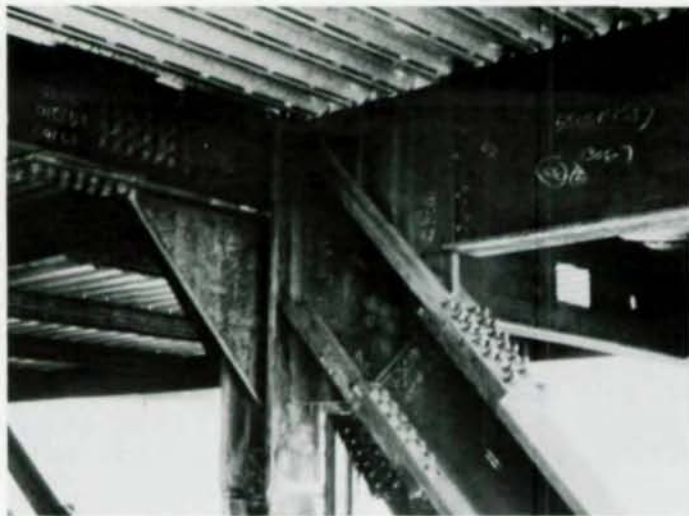
Fig. 8. Outrigger superdiagonals connected to vertical columns
