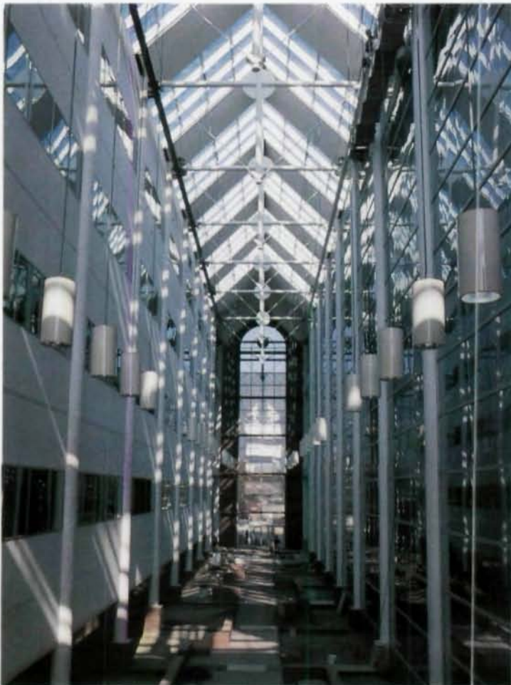
Handsome, Gothic-styled "spline" (above) connects new and existing buildings. Photos (r.) show spline's steel-framed construction.
