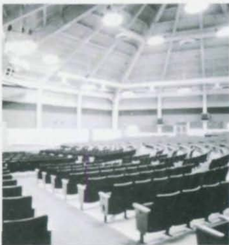
Clear-span (150-ft) auditorium seating 1,500 permits indoor race viewing and serves as walking ring and sales facility for thoroughbreds. Below (l.) shows interior seating arrangements. Below (r.) details steel framing of large pavilion.
