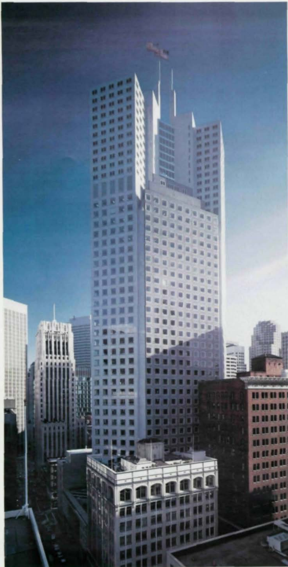
Steel-framed California Center was challenge in both design and site conditions.
