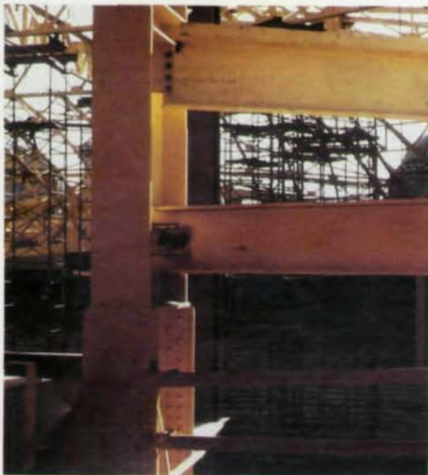
Detail of new column stub welded to existing column, which supports proscenium trusses to be attached on left side.
