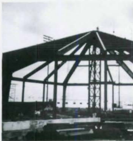
Clear-span (150-ft) auditorium seating 1,500 permits indoor race viewing and serves as walking ring and sales facility for thoroughbreds. Below (l.) shows interior seating arrangements. Below (r.) details steel framing of large pavilion.
