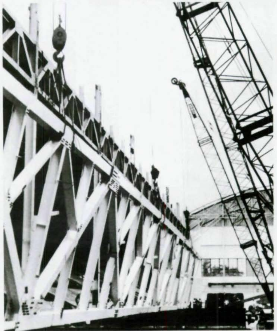
Fabricators assemble 240-ft trusses (above). Each weighing in at 21 tons, trusses were key to fieldhouse renewal. Three cranes lifted each truss in place (r.).
