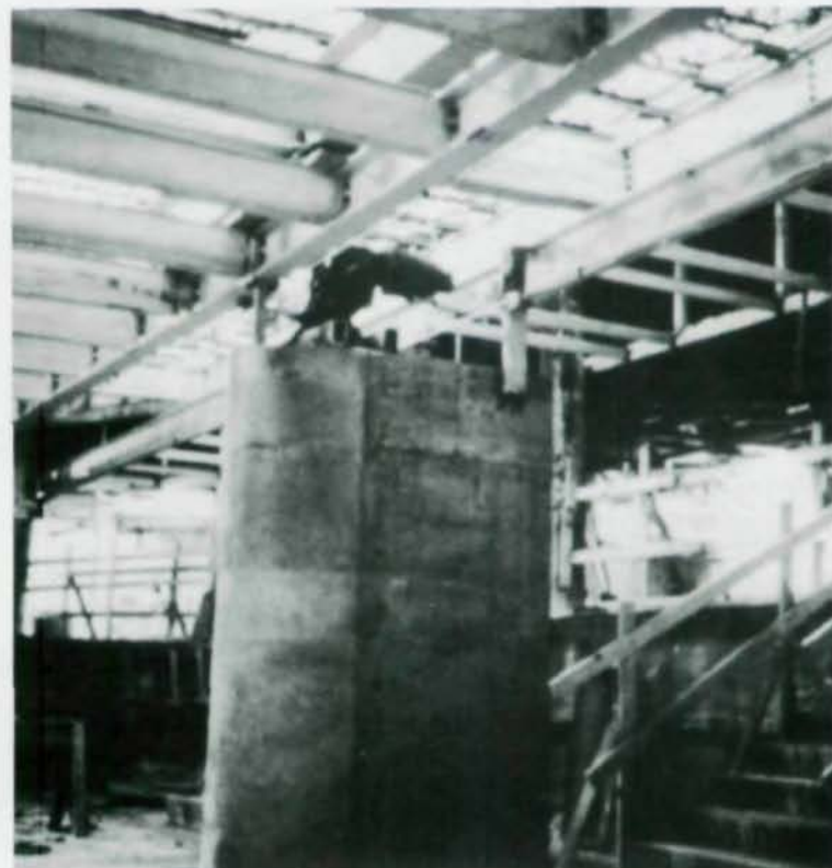
New tilting floor framing
