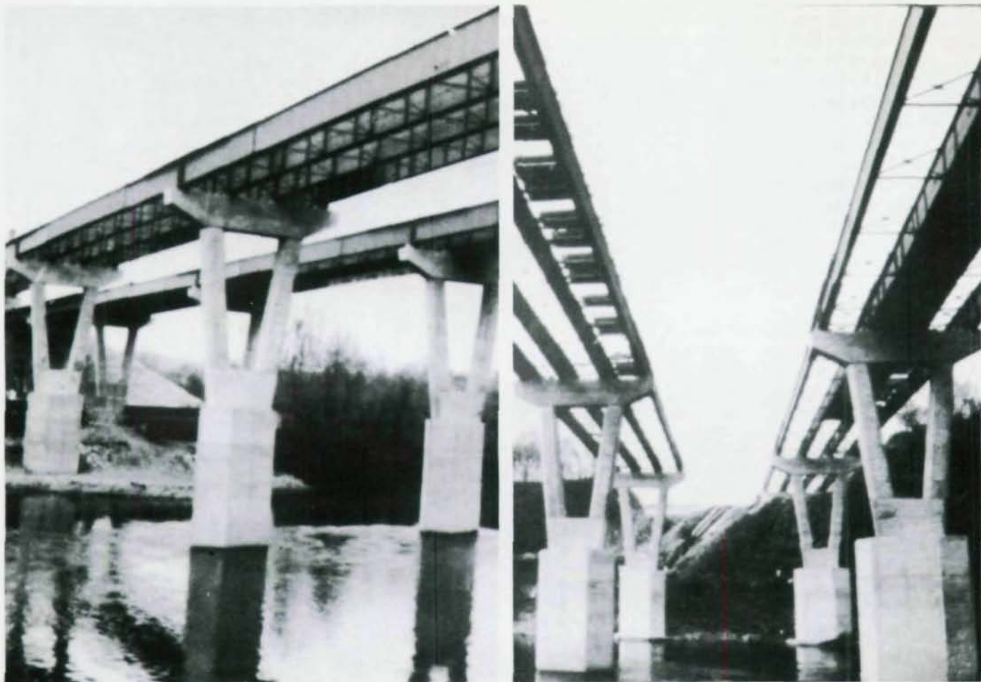
Two views of I-78 steel bridge.
