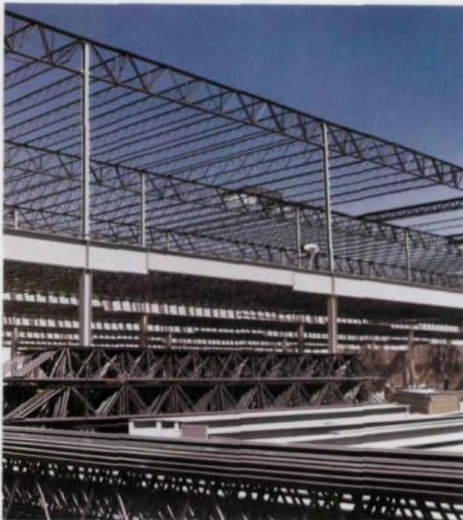
The simplicity and light weight of Vulcraft joists and joist girders make erection faster and easier.
