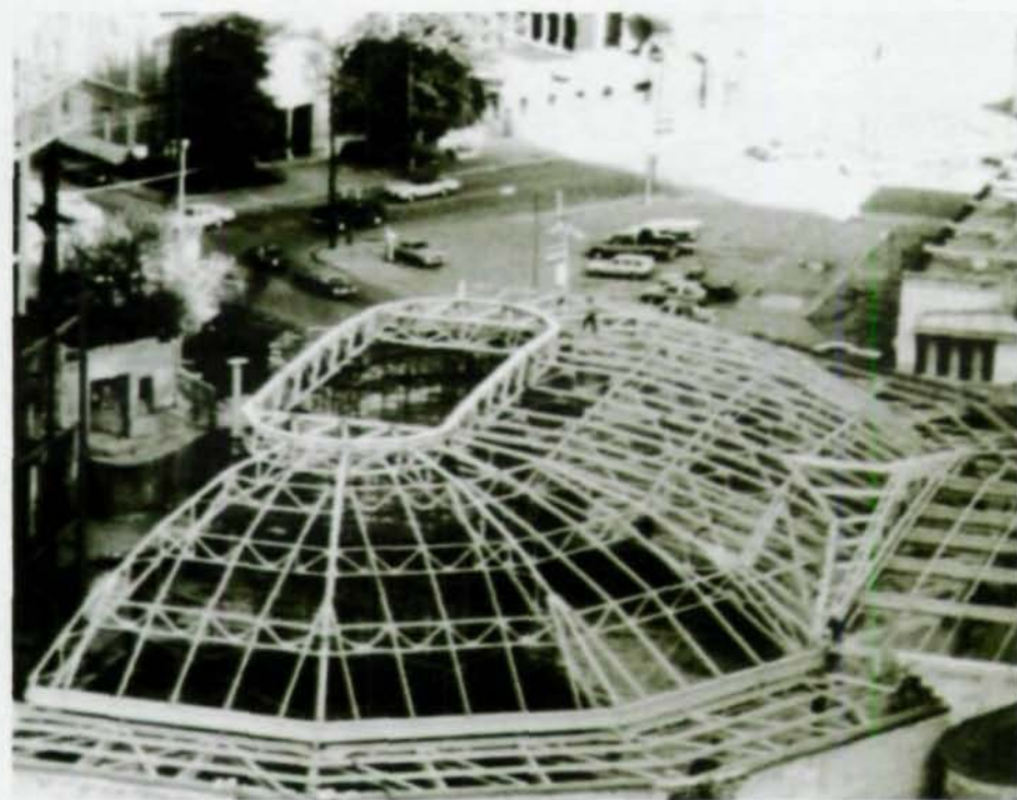
New dome under construction, with stage-house framing and temporary shoring on left.
