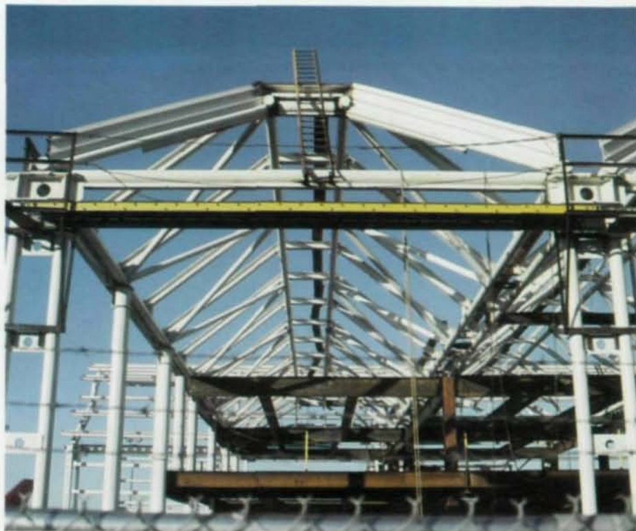
Folded-plate support detail at end fold (above). View of two-column cluster supporting folded-plate trusses at roadway side (r.)
