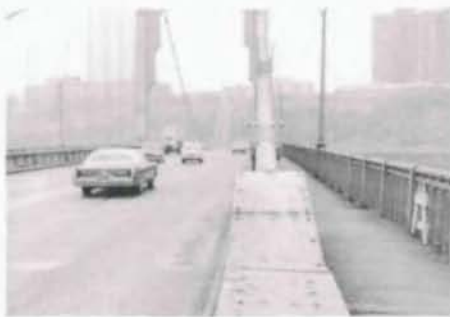
Fig. 2. 10th Street Bridge, Pittsburgh, Pa. Deck type, 3-in. tee, installed 55 yrs. At major rehab in 1981, deck was in excellent structural condition, overlaid with rubberized asphalt.
