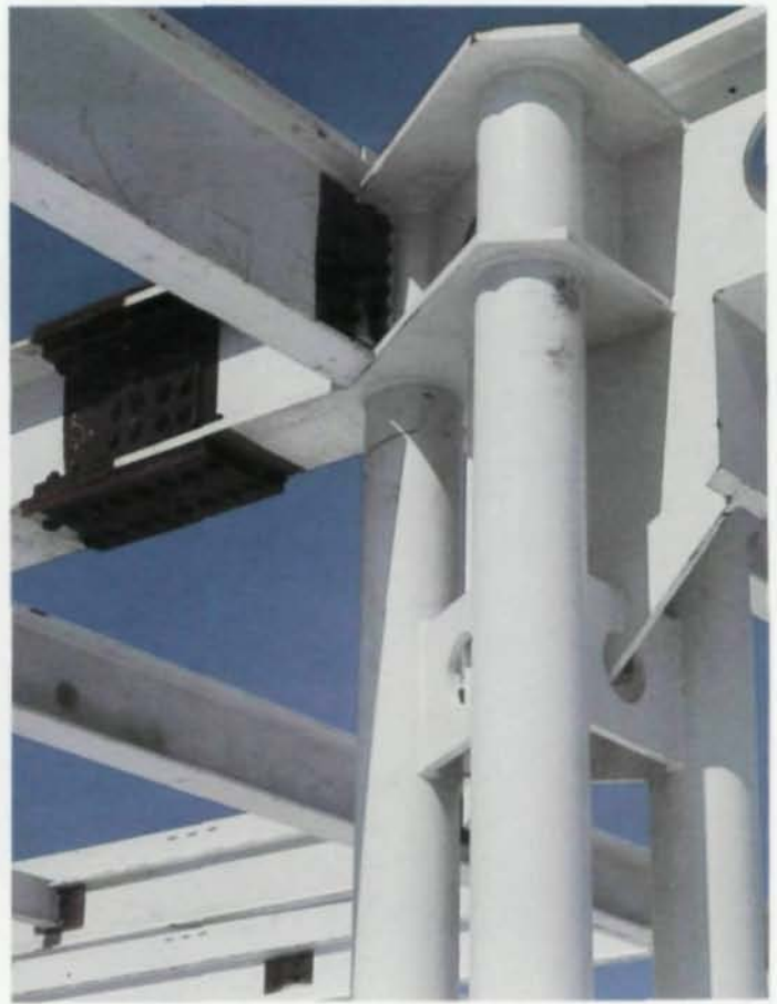
Vault to Vierendeel column connection Concourse C (3-column cluster)
