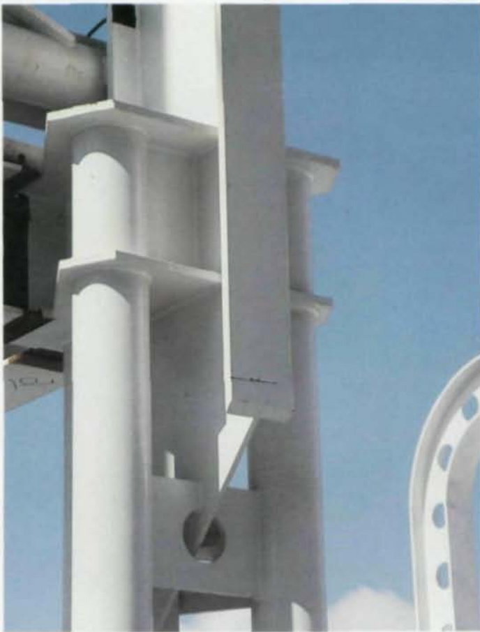
Vault to Vierendeel column connection Concourse B (3-column cluster)
