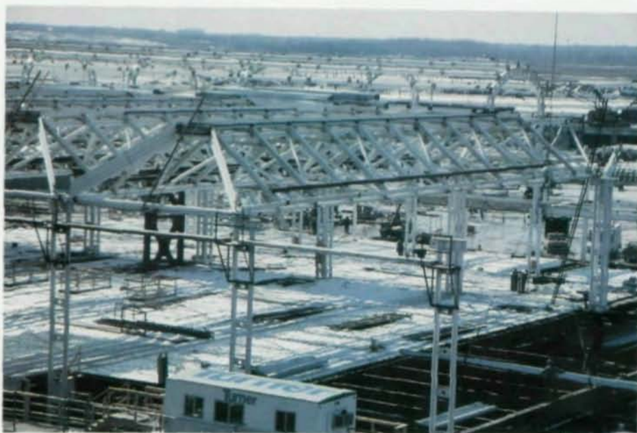
Unclad folded-plate trusses and struts
