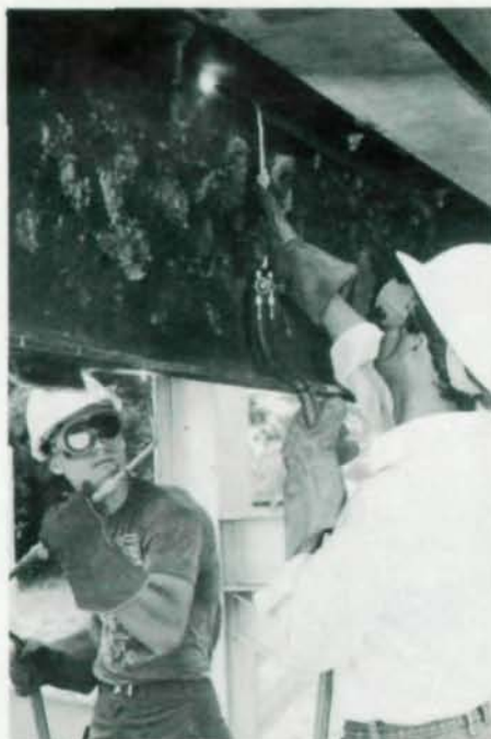
Tempering heat applied with torch.
