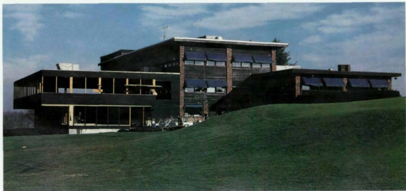
Steel framing was material of choice for Hawthorne Country Club addition.
