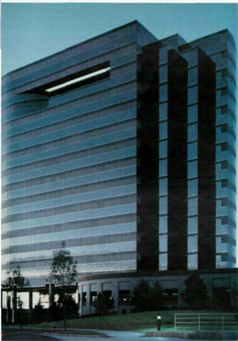
Orientation and elevation of building, layout of parking deck, grand lobby and views create design above usual "office park." Long, cantilevered beams form serrated building ends. Photo by Martin Cole
