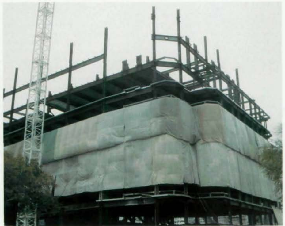
Fig. 4. At levels 2-10, tree-beam frames are at ends of tower.
