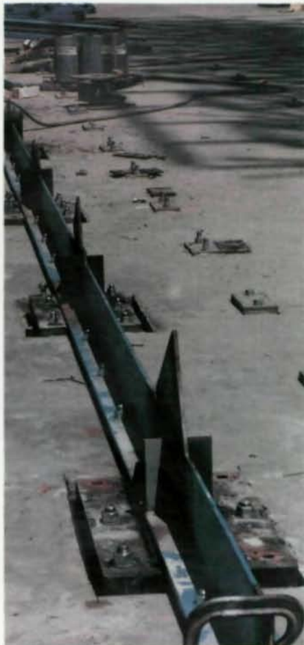
Collar plate condition at typical flue post (l.). Uplift base plate (r.) at ends of down-aisle frames.
