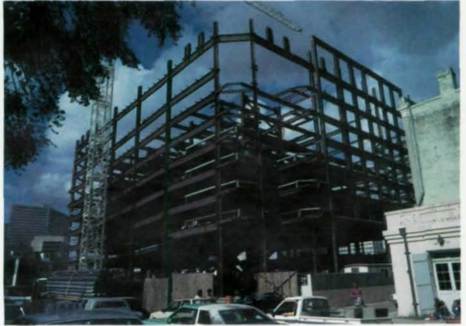
Fig. 4. At levels 2-10, tree-beam frames are at ends of tower.
