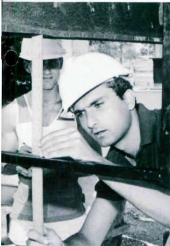
Repaired girder checked for alignment.
