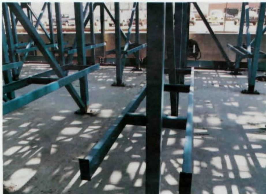
Sections of cross-aisle frames are field-welded in on-site welding jig.
