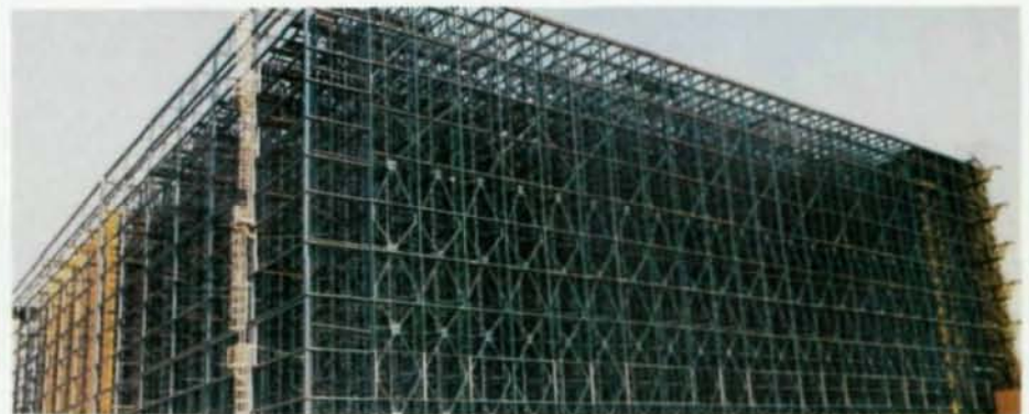
One of first rack-supported structures in California. Aerial (top) indicates size. Interior (c.) down-aisle view of braced-frame system. Long frames (bott.) are laterally stayed by cross-aisle frames.
