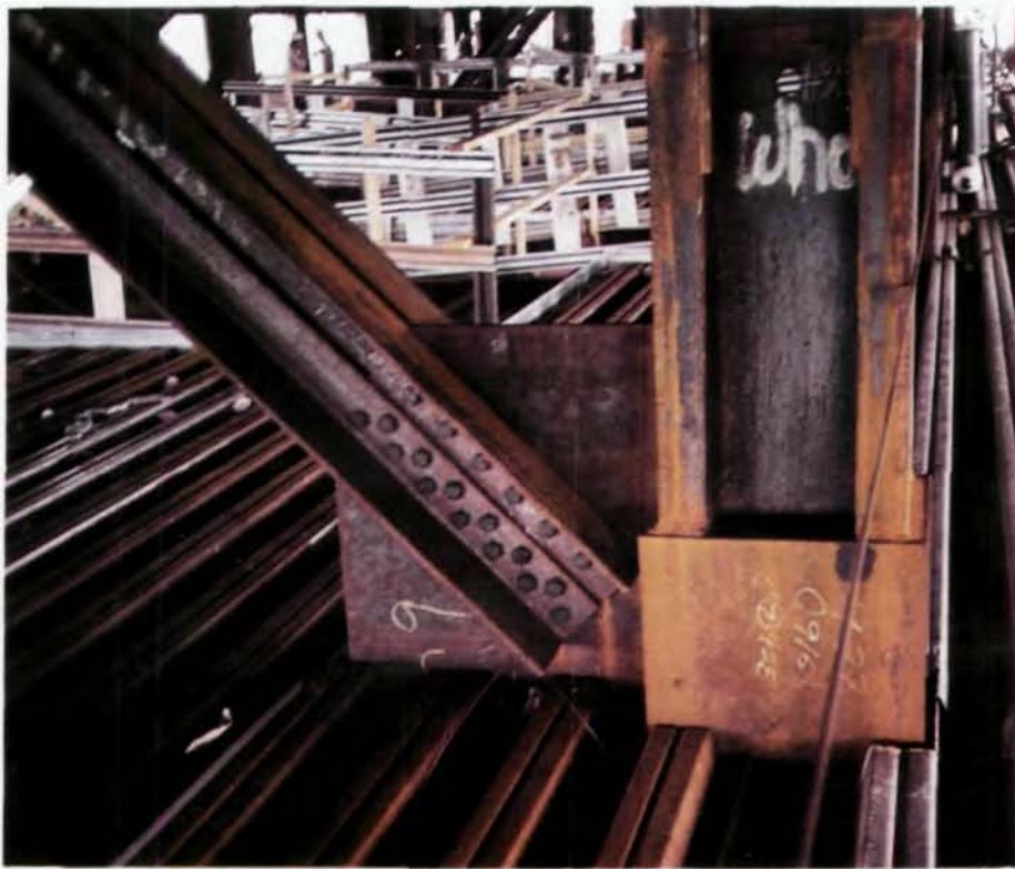
Single line of diagonal bracing used for wind resistance.
