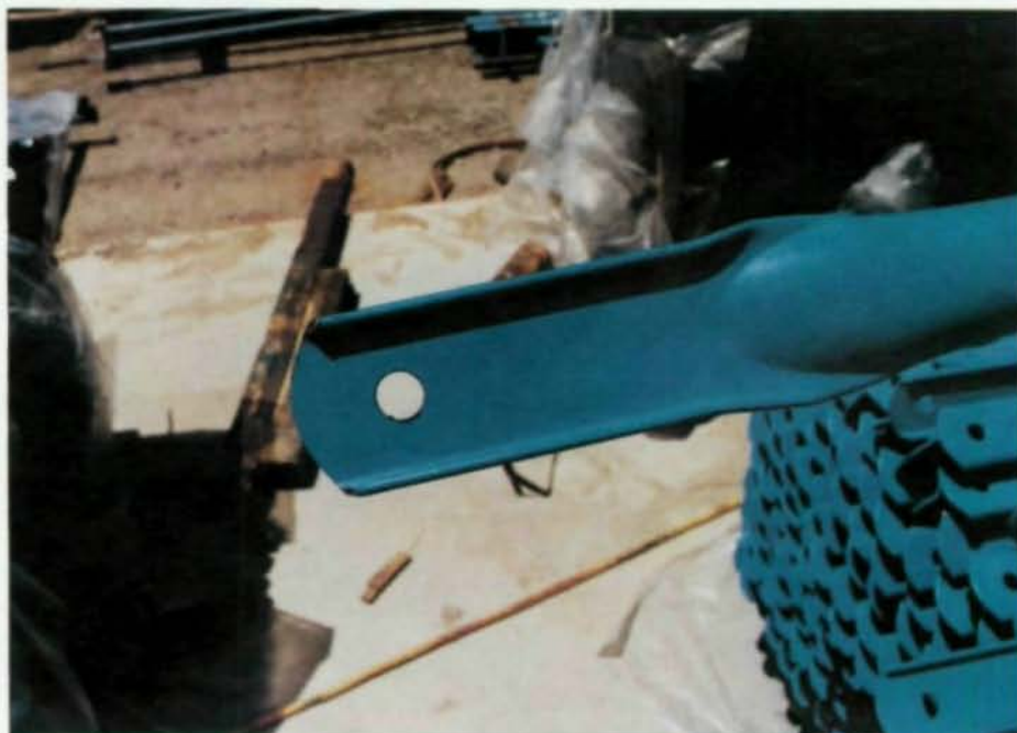
Fig. 4 (top). Post splice connection detail used to develop full tensile capacity of post. Typical pipe strut end condition (bott.).
