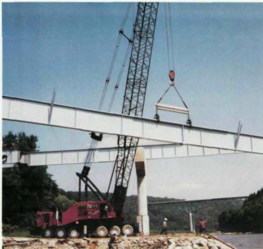
Comparatively light steel girder sections swing into place.
