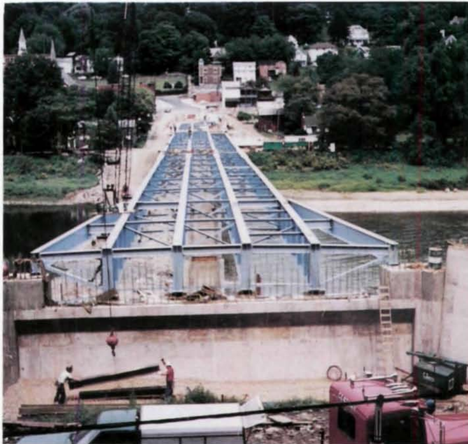
Clean, uncluttered steel frame of Emlenton Bridge superstructure
