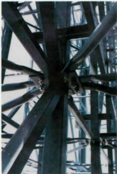
Post splice connection detail (l.). Installation of collar plates (r.) at typical aisle and flue post conditions
