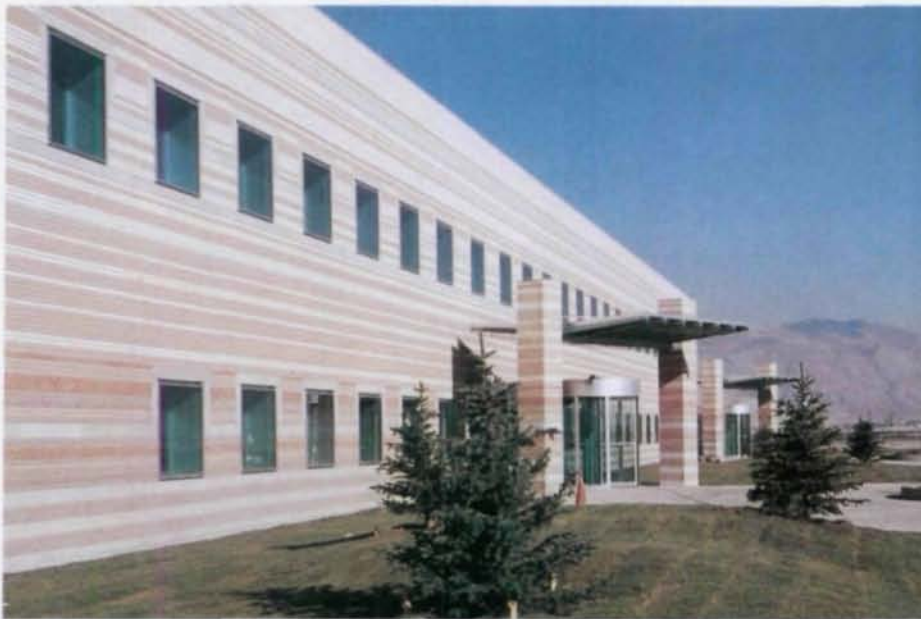
Exterior highlights layered brick coursing and triple-pane window treatments. Entry canopy and vestibules in background.
