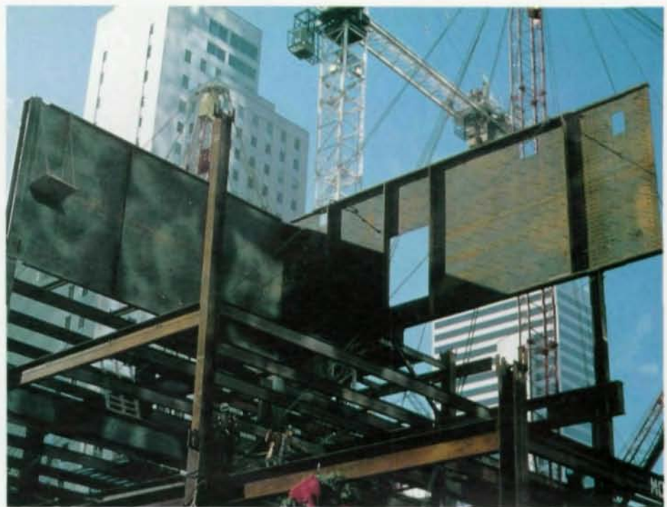
Construction photo shows level 6 transfer girders.
