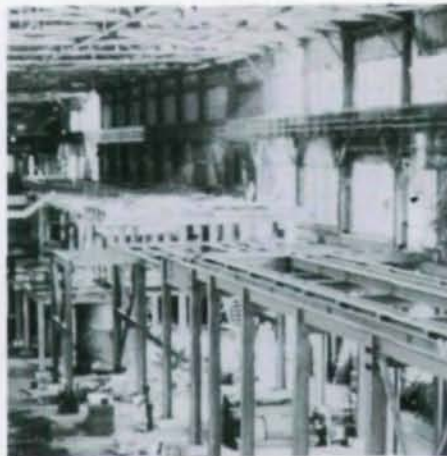
Existing process control building framing (l.). Electrogalvanizing line frame before equipment installation
