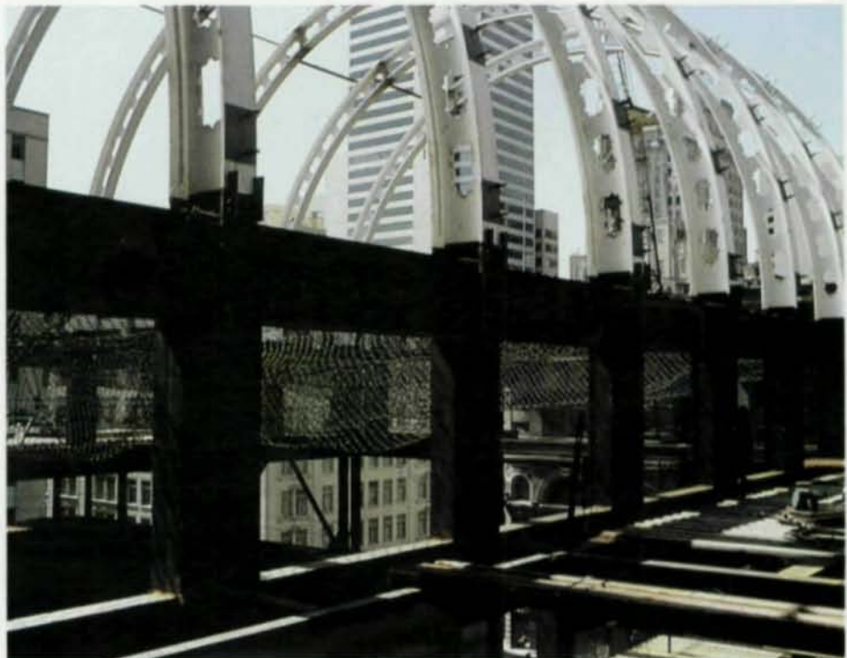
Construction photo shows banking hall roof framing.
