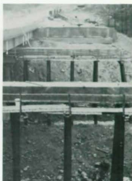
Move complete, ready for superstructure removal
