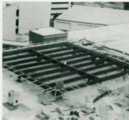
Steel framework erected and large pre-welded panels support safety net. Ramp (bott.) leads directly from helipad to hospital.
