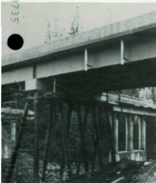
New superstructure ready for permanent piers
