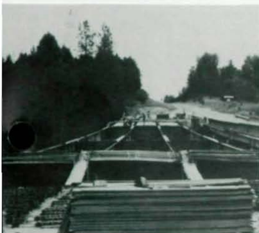
New girders in place, ready for decking
