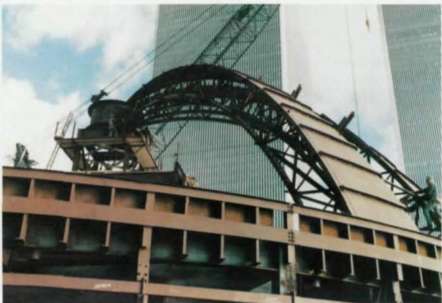
Steel-framed dome tops World Financial Center. Entire "slice" (r.) was lifted into place and connected to tension ring and compression hub. Process was repeated—650 ft up—until dome was completed.
