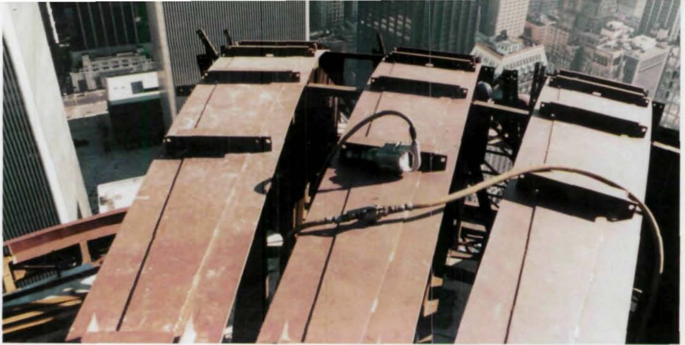
Gaps between arch-truss assemblies were filled in with curved plate segments welded in field.
