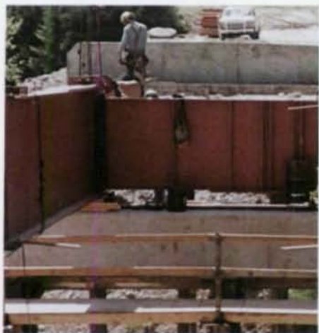
Steel set on temporary substructure
