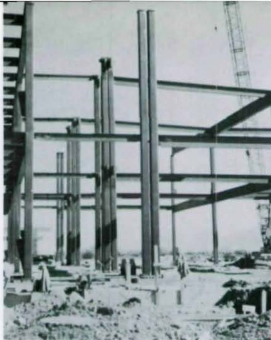
(L. to r.): Diagonal steel tube braces permit regular spacing of windows. Double columns along exterior create center expansion joint. Circular cutout for main lobby.
