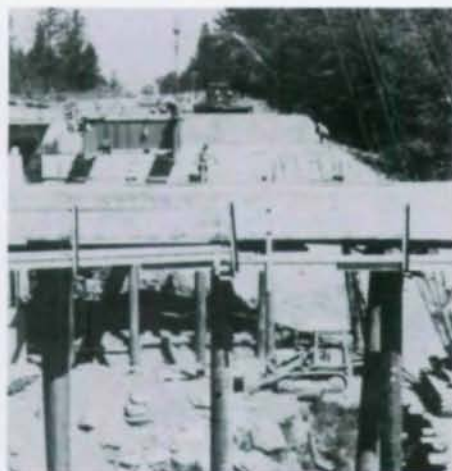
Steel set on temporary structure
