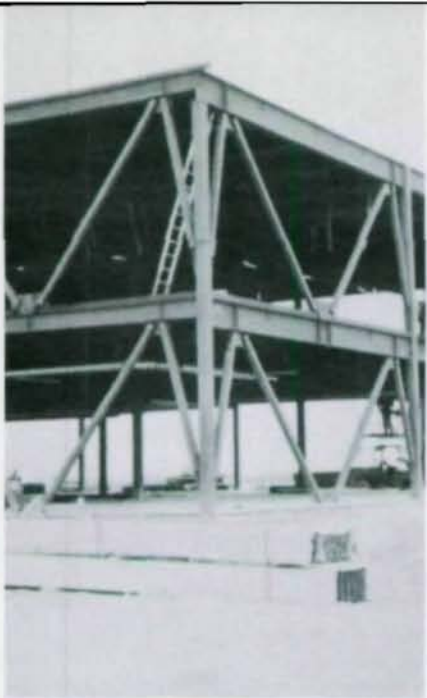
(L. to r.): Diagonal steel tube braces permit regular spacing of windows. Double columns along exterior create center expansion joint. Circular cutout for main lobby.
