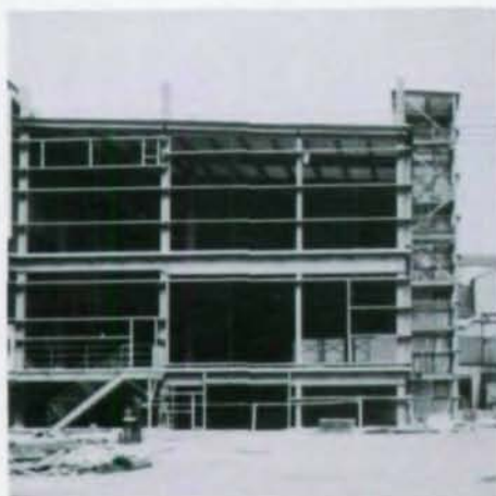
Existing process control building framing (l.). Electrogalvanizing line frame before equipment installation
