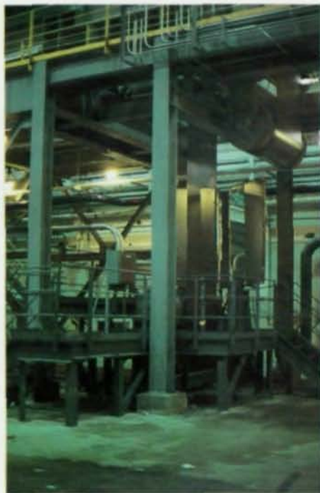
View of inspection station
