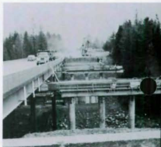
Air winches pull superstructure over
