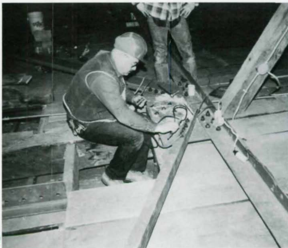
New tubular steel framing (above) supports old wood beams. Below, connections are bolted on attic truss (no welding permitted).
