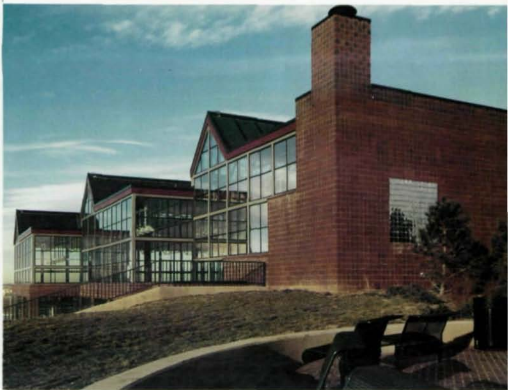
Exterior of pool wing shows high, two-story walls of non-fogging glass. Ed Leland photo.
