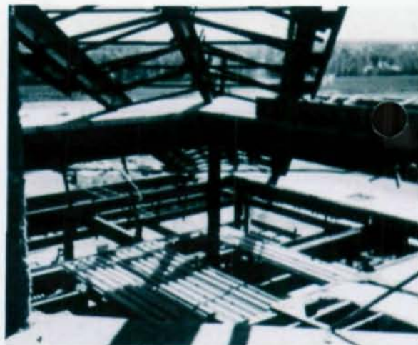
Photo shows steel spline framing where sides of pyramid meet.
