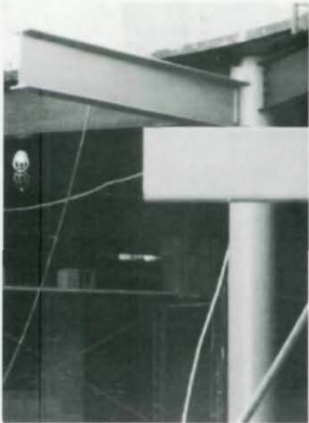
Section through stair detail of cantilever beam support for stringers (above). W14x30 and tube sections cantilever off 10-in. pipe columns (r).
