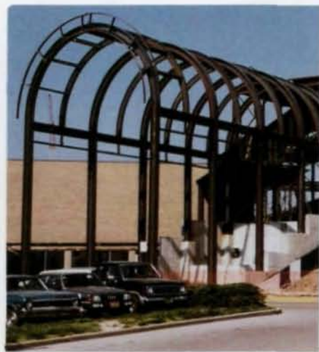
St. Ann's Entrance, with arched steel canopy, under construction
