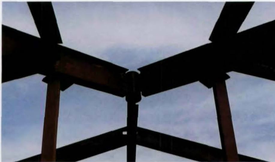
Core intersection, with pipe collar to ease fabrication of ridge/valley connections.
