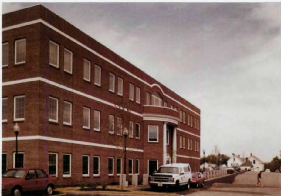
Exterior of new facility designed to fit maritime feel of area. LRFD design proved cost-effective.
