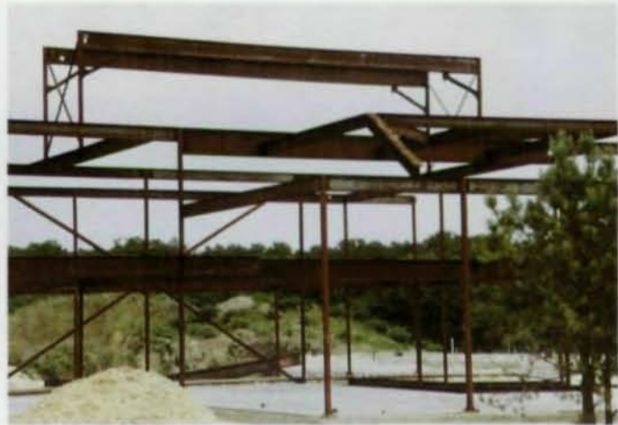
Residential courtyard looking toward dining room (above). Second floor and roof steel-framed for dining room and cathedral ceiling.
