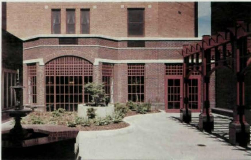
*The large setbacks, combined with the decorative exposed steel, breaks up Canterbury Place's huge mass and allows it to better meld with the surrounding community. Exposed steel is used in a variety of ways on the project, including the prote cohere/entrance, trellised walkway, upper level wind and sunscreens, and for the steel-framed windows.*
