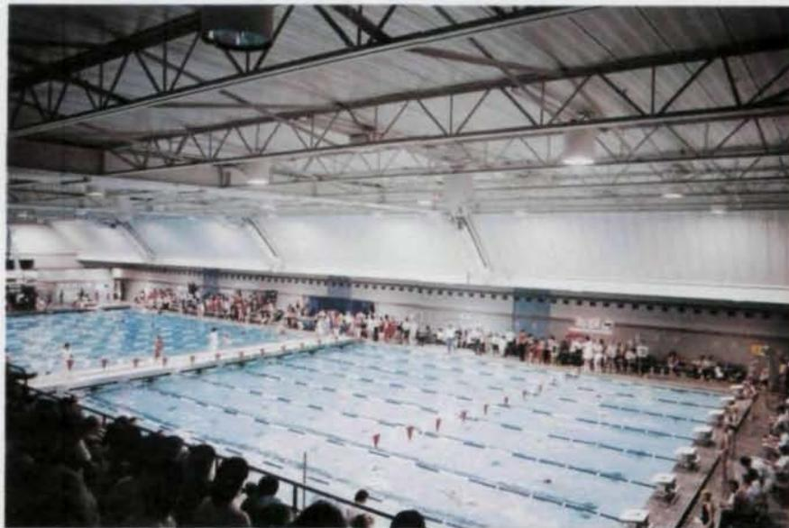
wouldn't use them for beams, except where they're exposed or in a food processing plant [where health codes require the elimination of ledges that could cause food contamination]," Kloiber said. "They're not as efficient in bending as an open shape, and the connection cost is higher. They do work well for torsional problems, and they work well where an attractive appearance is necessary."
