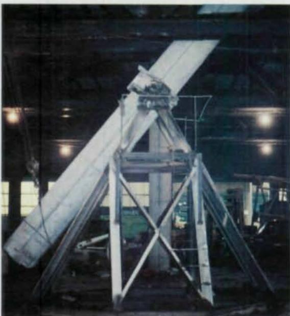
*Crossbracing (above) was installed on each end of the span to tie each pair of trusses together.*
