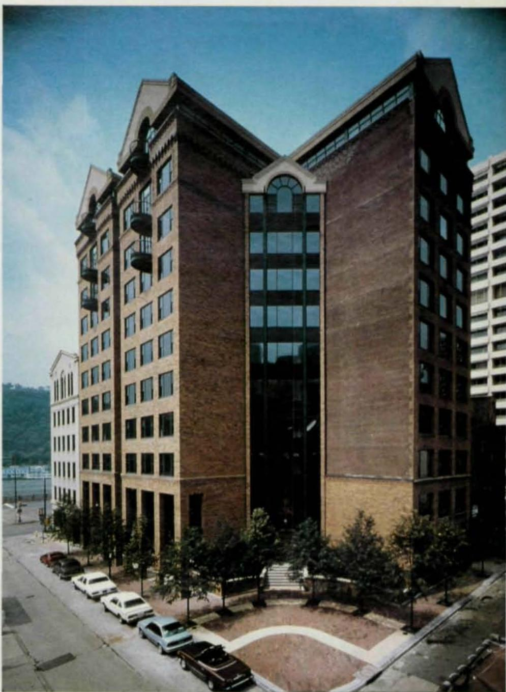
*A 28,845-sq.-ft. addition was constructed as part of the renovation of the former Shields Rubber Co. Warehouse into a modern office building. The use of a lightweight steel frame was essential to match the floor heights of the existing building and to provide the desired 35' on center bay spacing. Construction photography by Fred P. Kenderson; finished photography by Maurcen Wikiera.*
