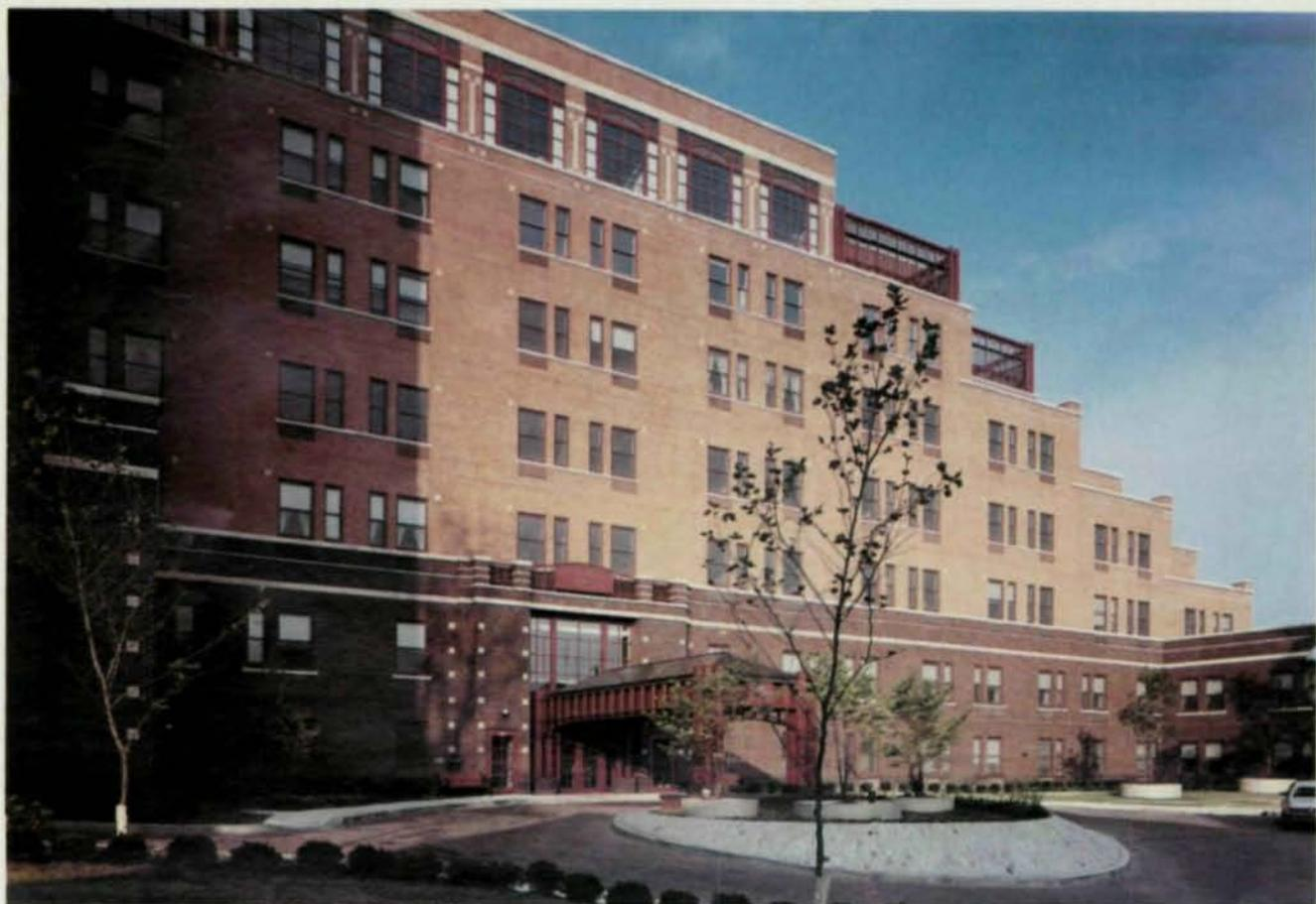
design, it also created headaches for the structural engineers. "The setbacks don't occur at the normal bay spacing, so there was no way to introduce a bearing partition at that point," said Gilbert Kaufman, an engineer with Structural Engineering Corporation, Pittsburgh. In addition, each level features more than one setback.
