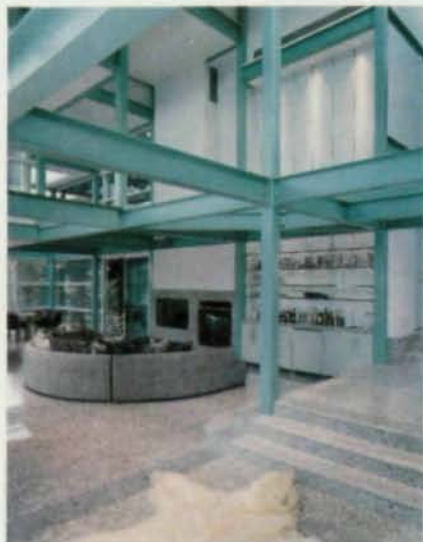
Steel was left exposed on the inside in order to give visitors an understanding about the methodology and construction of the home.
