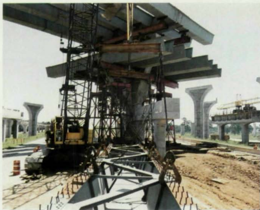
A massive tree pier rises 80' at the heart of the interchange.
