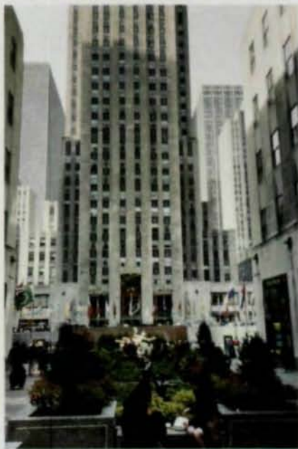
A new central refrigeration plant was installed in New York's GE Building.
