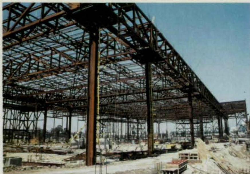
Each column supports a pair of 20'-deep transverse primary trusses and a pair of 20'-deep longitudinal secondary trusses.
