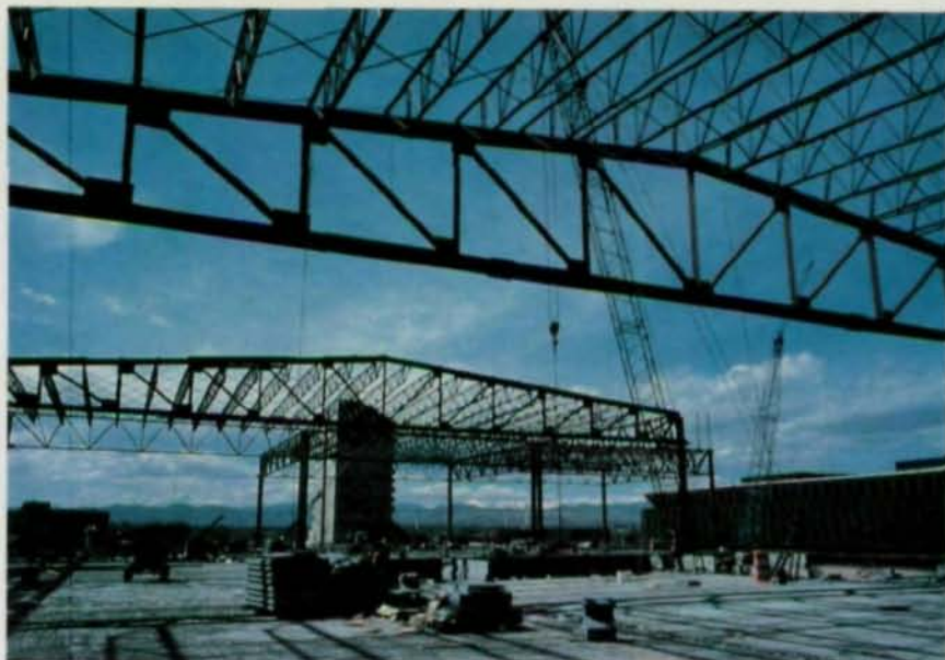
The tight construction schedule mandated the erection of one truss per week. Using two crews, each truss took two days to field splice together and another six hours for two cranes to hoist into place.
