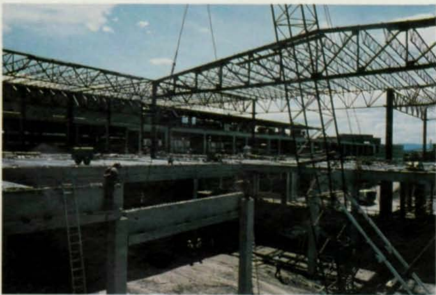
The $126 million Denver Convention Center includes 300,000-sq.-ft. of exhibit space on the second level. The exhibit space sits on top of a large ballroom and is supported by seven jumbo trusses, each 12'-6" deep and 150' long, with the heaviest weighing 135 tons. Opposite page photo by Nick Merrick of Heidrich Blessing.
