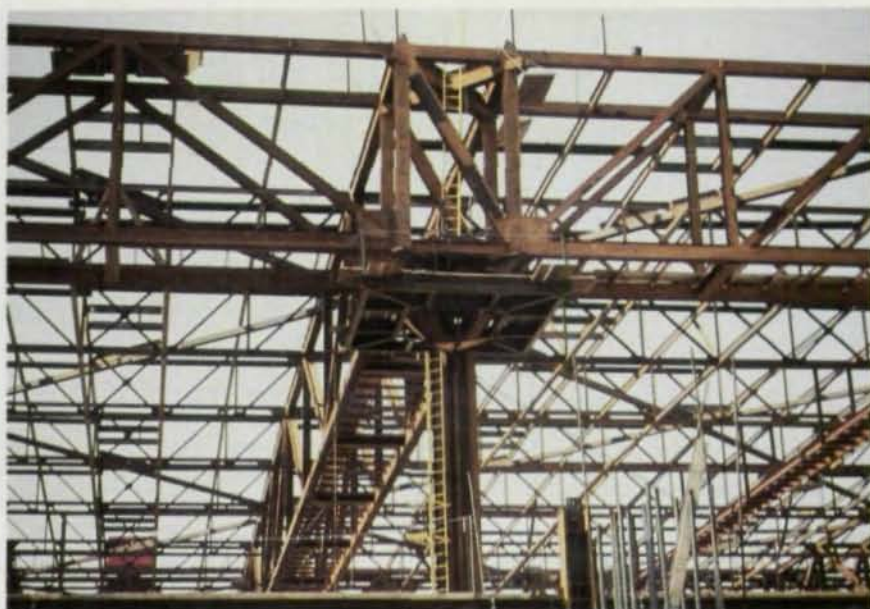
The roof of the giant exhibit hall is supported on a series of trusses, which in turn sit on steel "tree" columns. The columns are built up into a cruciform shape and consist of four 14" wide flange shapes welded together around a 16"-square central tube.
