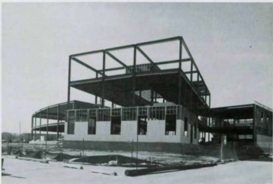
Construction photography by Bernstein Associates.
