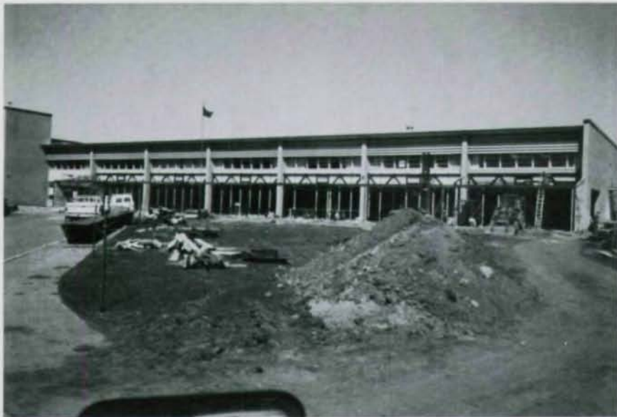
...a new steel truss was added to carry the load supported by the I-beams...
