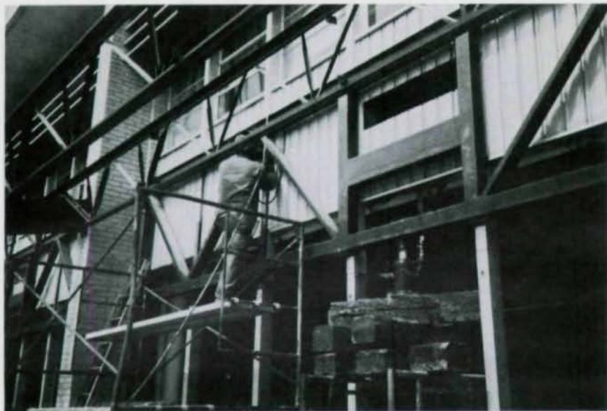
...the truss consists of rectangular steel tubes...
