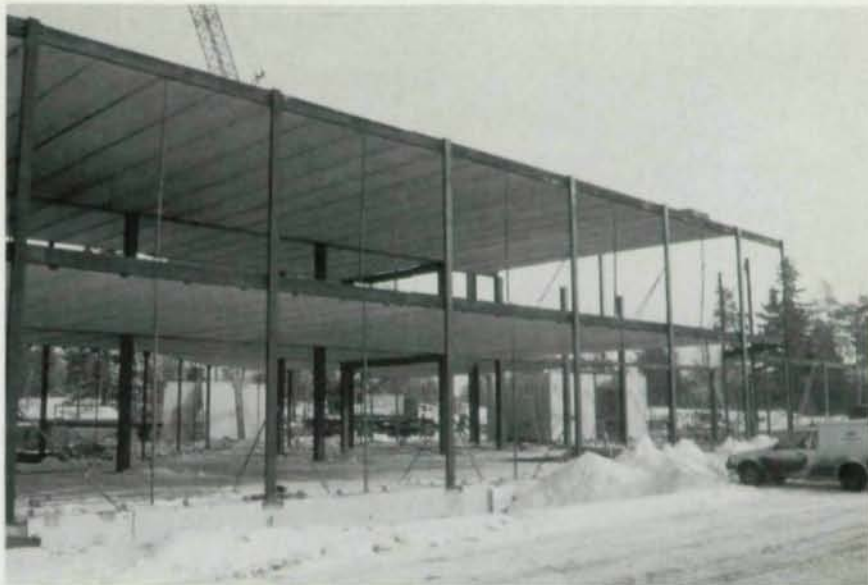
The system of through columns and simply supported beams, such as on this low-rise office building in Stockholm, can easily accommodate dimensional deviations and has become the dominant system in Sweden.
