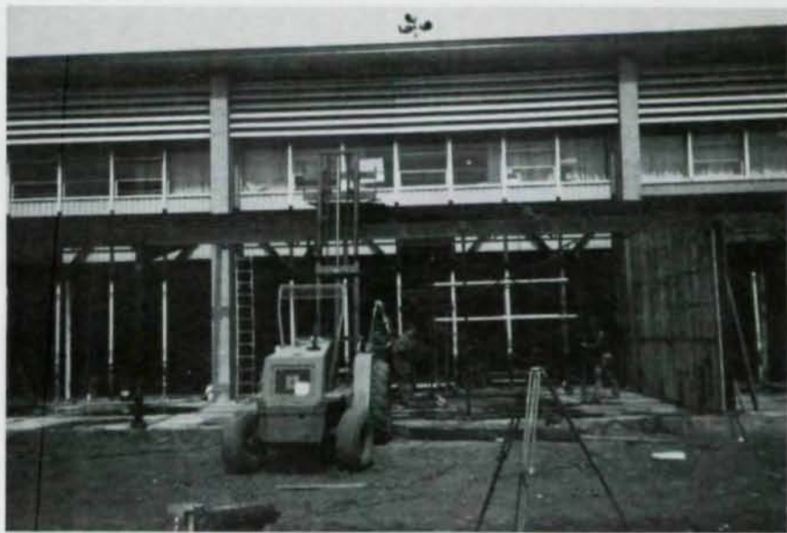
...while the new construction consists of open web steel joist purlins supported primarily on steel stud bearing walls...
