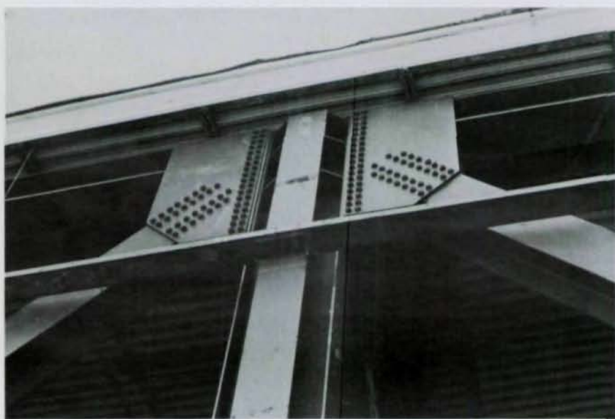
Slender vertical pipe hangers and diagonal rods were used to support the elevated track, which eliminated the need for support columns that would have interfered with the column-free nature of the lower level (top). The use of bolted connections helped to enhance the visual character of the structure.
