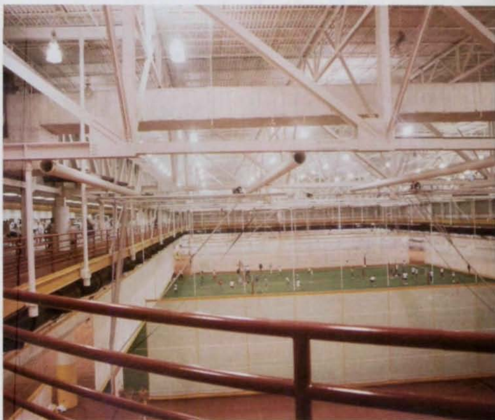
The steel structure of Iowa State University's new recreation center was left exposed both to reduce costs and to add visual texture to the space. (Construction photo by Person Studio)
