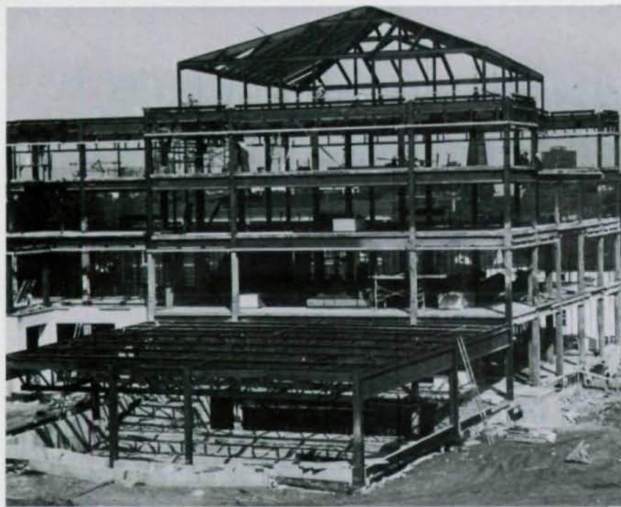
The design of a two-story gallery in the middle of the Lehigh University's new Business School required that girders be discontinuous in that area. In that area, the roof is the only structural link.
