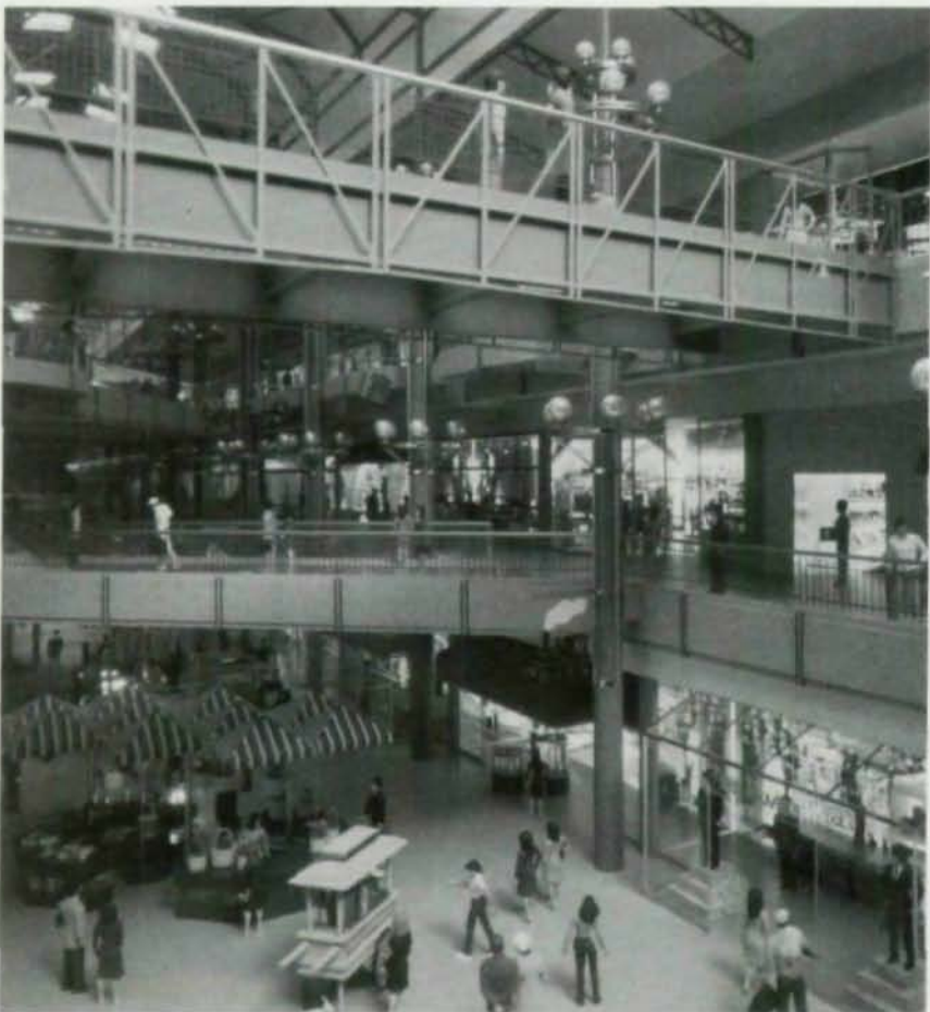
Exposed steel is used throughout the project, as illustrated in this model photograph (bottom). West Market, for example, will feature exposed steel bow trusses, joists and joist girders supporting a barrel vault metal roof deck.
