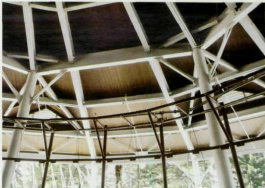
Since the roof consists of pie-shaped sloping segments, special girders were designed to receive the multiple ridge beams that supported each segment.
