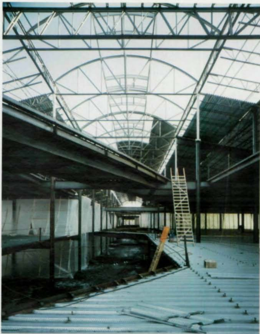
The bow trusses in West Market street will be exposed as an integral part of the architecture. The steel roof trusses in Knott's Camp Snoopy frame into the Vierendeel columns with moment connections in both directions providing lateral stability. Photographs by Peter Renerts.
