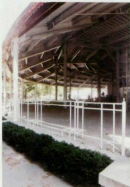
Since the roof consists of pie-shaped sloping segments, special girders were designed to receive the multiple ridge beams that supported each segment.
