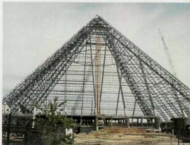
PYRAMID ARENA Consulting Engineer: Walter P. Moore & Associates; General Contractor: Huber, Hunt & Nichols, Inc.; Steel Fabricator: Havens Steel; Erector: Barnhart Construction Co.
