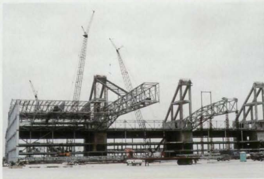
Great care was taken during the design and erection of the steel members. The erector, Derr Construction Co., lifted the box section in three parts and provided three sets of shoring towers to temporarily support the box sections prior to adding the tension struts.
