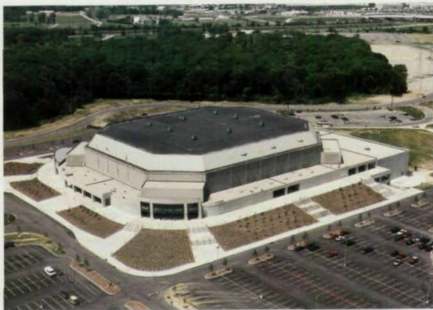
The mansard-style roof shape reflects the original structural design of the center. When that system proved too expensive, the engineers switched to a more conventional steel system but managed to still keep the aesthetically desirable roof shape. Photo by Greg Girard
