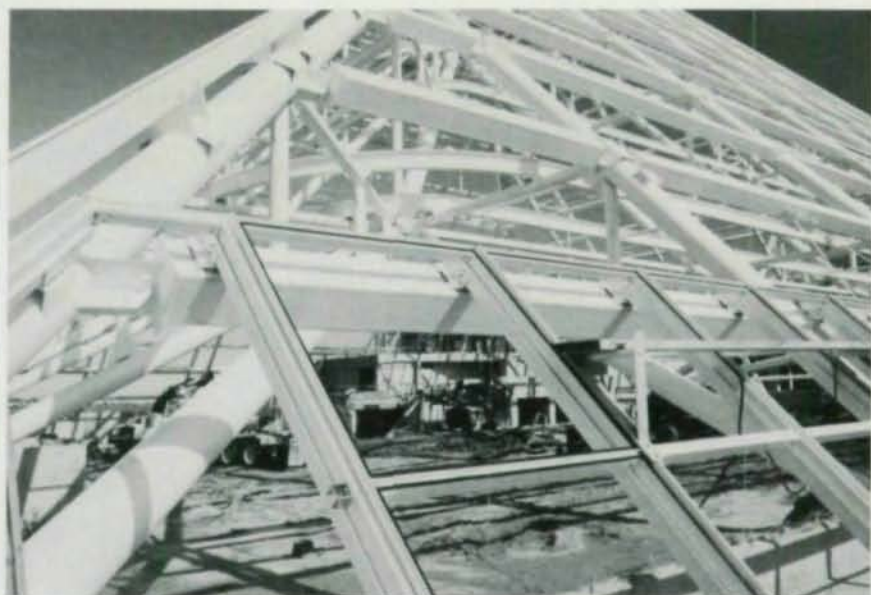
Shown above is the start of the glazing mullion installation at the base of the pyramid.
