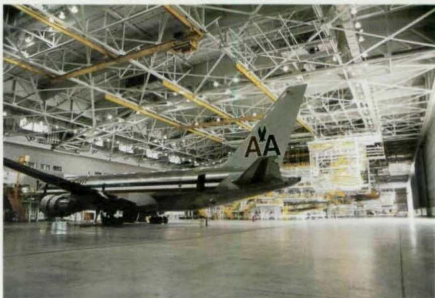
The inside of American Airline's new maintenance and engineering facility is designed without columns to accommodate even the largest aircraft. The roof structure can support 540,000 lbs. per bay.
