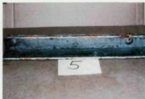
An angle from the steel bridge railing of the Ewing Park Bridge in Ellwood City, PA, in "as received" condition.
