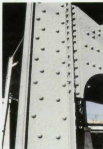
A close-up of riveted structural steel on the Swinburne Bridge in Pittsburgh after "upgrading".
