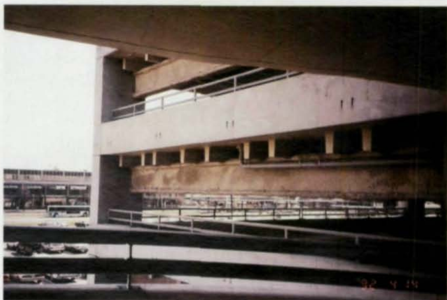
A structural steel superframe with untopped precast concrete double tees was the most economical system for a new parking structure at JFK International Airport in New York.
