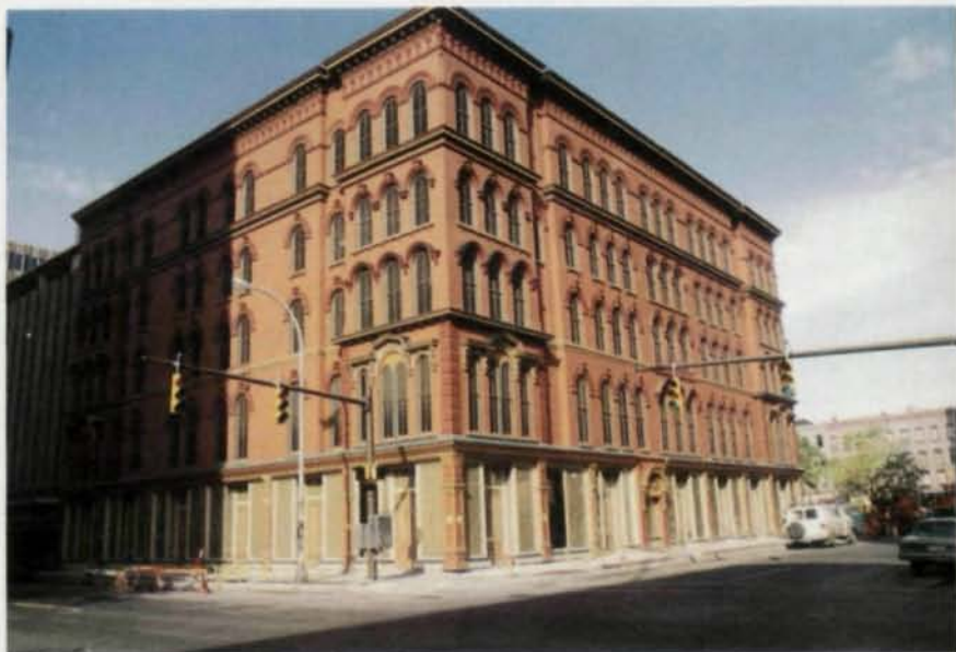
The historic Larned Building in downtown Syracuse was reborn as a steel-framed parking structure through an innovative and difficult construction process.
