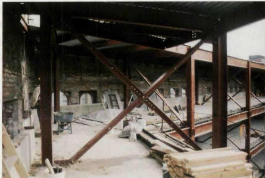
The steel frame's X-bracing was located so as to not interfere with either parking or vehicular traffic.
