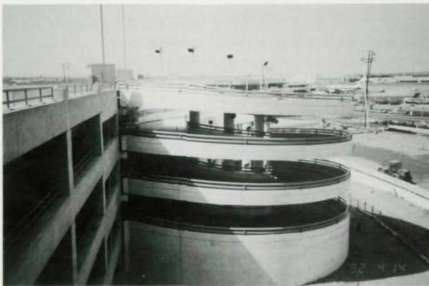
The parking structure features a double line of Grade 50 steel columns and beams spaced 3' apart, with the columns ranging in size from W14 x 176 to W14 x 605. The two external spiral ramps allow vertical circulation to each level of the parking garage. Each ramp has a one-way, counterclockwise travel direction.
