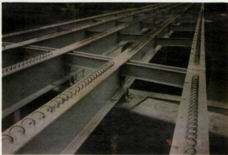
A closeup photo of the bridge during construction shows the new bottom plates.
