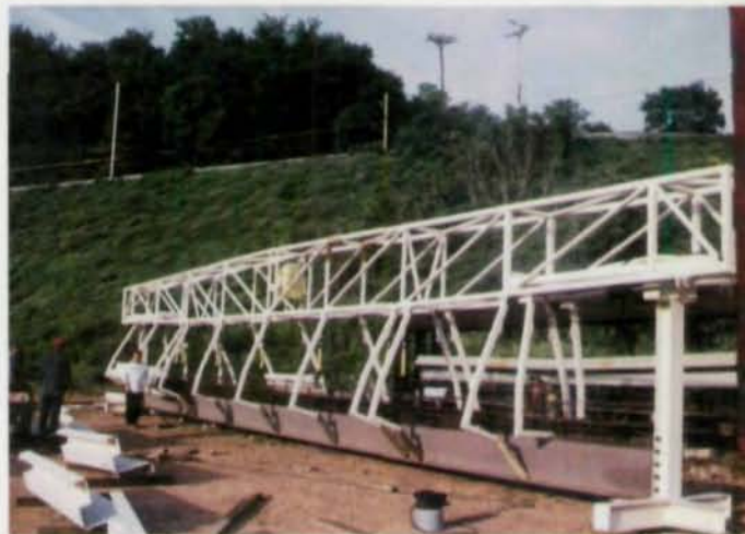
Shown above is the installation of steel side forms for the custom form of a composite system. Note a steel beam is already in position to receive the concrete flange.
