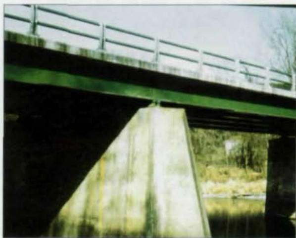
A retrofit project eliminated expansion joints in part by splicing the bridge's stringers.
