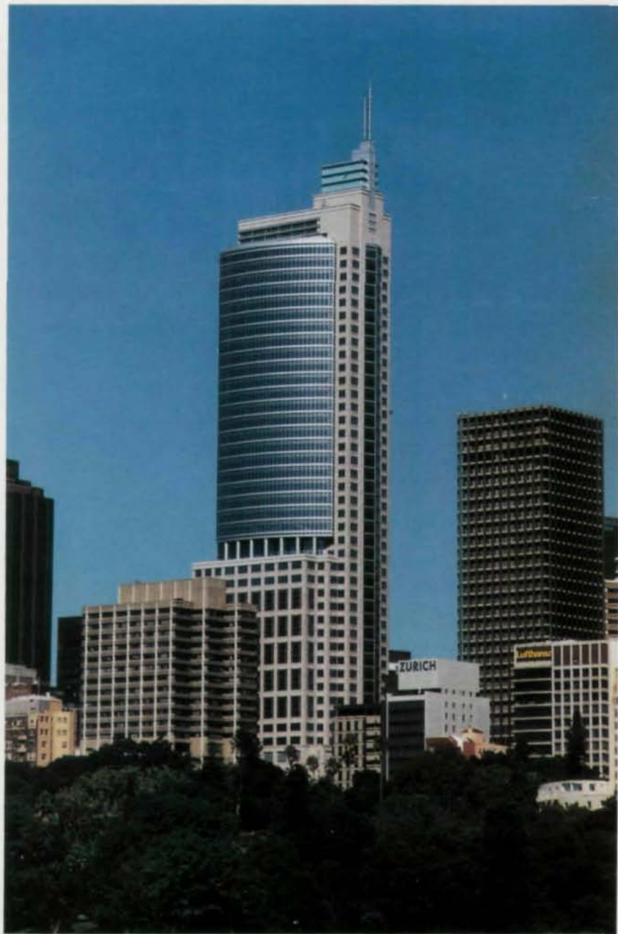
The Chifley Square Building facade is highly articulated to help create a transition from the local street front lines to the overall city grid, while also enhancing views of Sydney Harbour.
