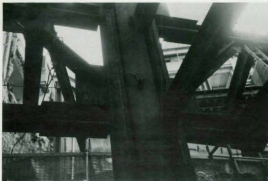
The basement core column shown above is built up from seven plates, while the split columns shown at right straddle a sidewalk arcade below.
