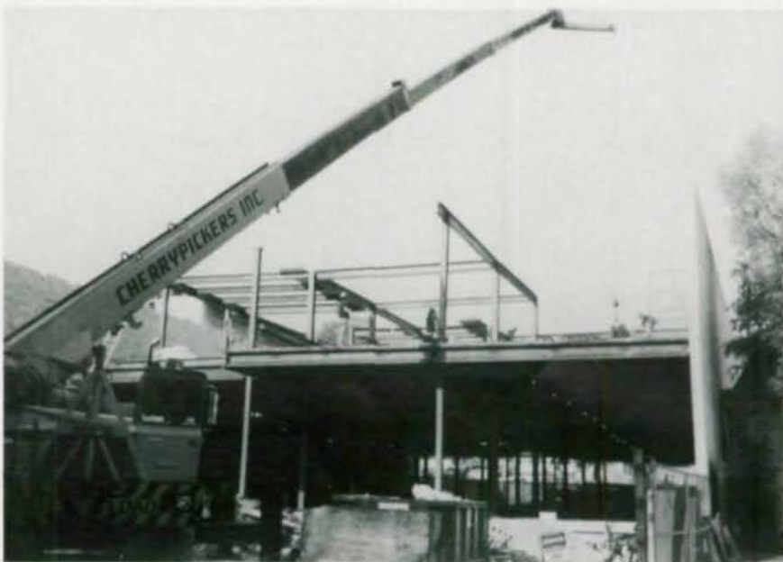
By using composite construction with partially restrained connections, the project's designer reduced the typical girder size from W14x34 to W14x22. The RGS design also reduced the number of studs required, though it did require the member to be cambered.
