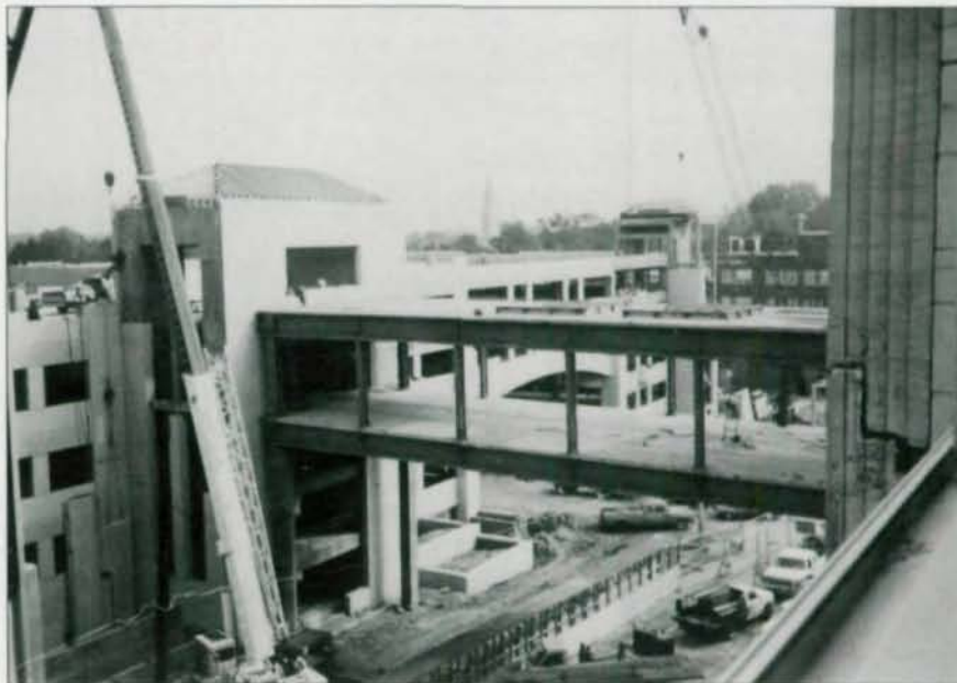
The designers chose a 30' x 30' bay size to maximize flexibility, including the possibility of adding an office or hotel tower. The construction also included a covered, 32'-wide pedestrian bridge that was framed at each side with coverplated W36x300 girders.
