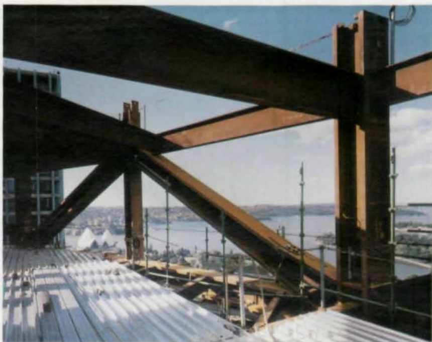
The transfer truss pictured above is located at one of the many setbacks with a view of the famed Sydney Opera House and Sydney Harbour. The core columns shown at left have bracing gussets with extended bottom plates for ease of erection. Note that the bracing connection plates stop short of the column face. Also, note the narrow rib deck.
