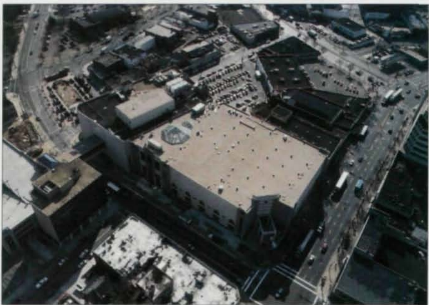
These two views show both the existing center and the new addition. Photo by Air Survey Corp.
