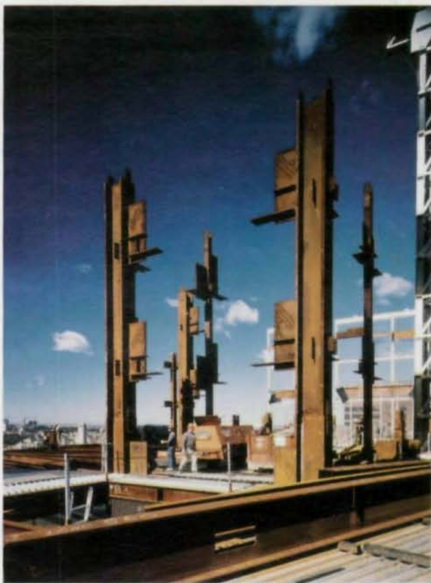
The transfer truss pictured above is located at one of the many setbacks with a view of the famed Sydney Opera House and Sydney Harbour. The core columns shown at left have bracing gussets with extended bottom plates for ease of erection. Note that the bracing connection plates stop short of the column face. Also, note the narrow rib deck.
