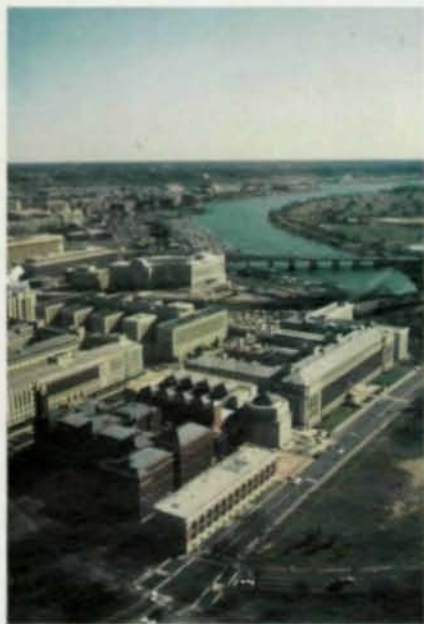
Shown on the opposite page are close up views of the turnbuckle bridges and the exposed steel Hall of Witness skylight (photos courtesy of Pei Cobb Freed & Partners; drawings courtesy of Gustavo Amaris, Weiskopf & Pickworth). Shown above is a daytime view of the museum with Washington, DC, in the background (photo courtesy of Jou Min Lin, Pei Cobb Freed & Partners).
