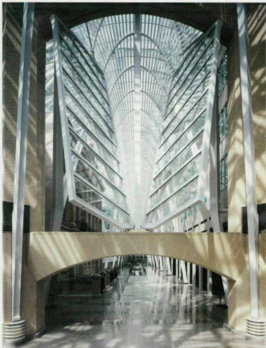
Separating the Galleria from Heritage Square is a large kinetic sculpture supported on a brick-clad steel beam. The large "windows", which pivot on a diagonal steel pipe, are framed with 6" x 6" hollow structural sections while steel tees are used for the horizontal elements. Photo by Robert Burley/Design Archive.
