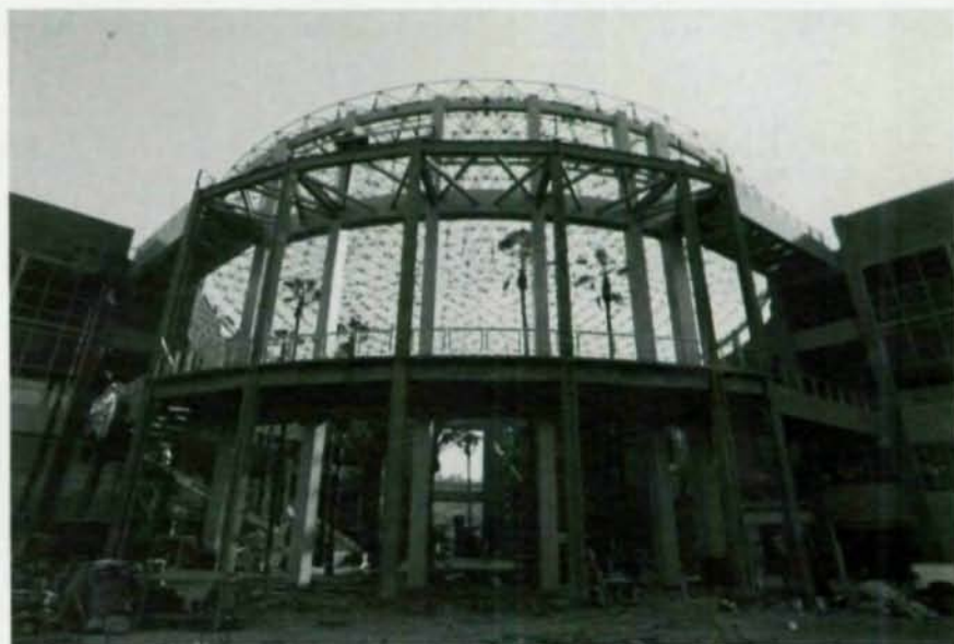
Steel was used on the project in order to achieve the tall forms and irregular shapes desired by the design team.
