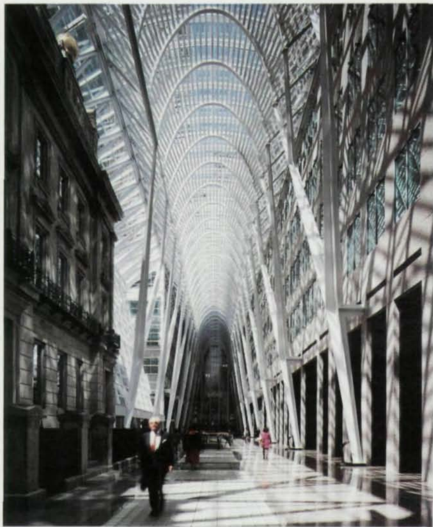
The steel columns and trusses at the Galleria in Toronto's BCE Place are designed to be symbolic of a country path surrounded by maple trees. Photos by Robert Burley/Design Archive.
