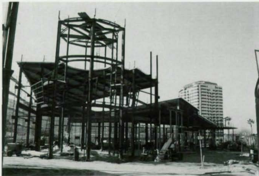
An Ordinary Moment Resisting Space Frame was used on this project for several reasons, including the high floor-to-floor heights and the many skewed connections and flying beams.
