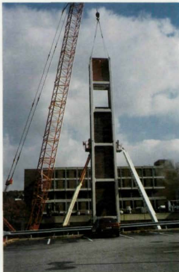
The composite view (opposite page) shows the completed boiler stack and its relationship to the existing hospital buildings and other new construction. Pictured at left is the stack addition under construction.
