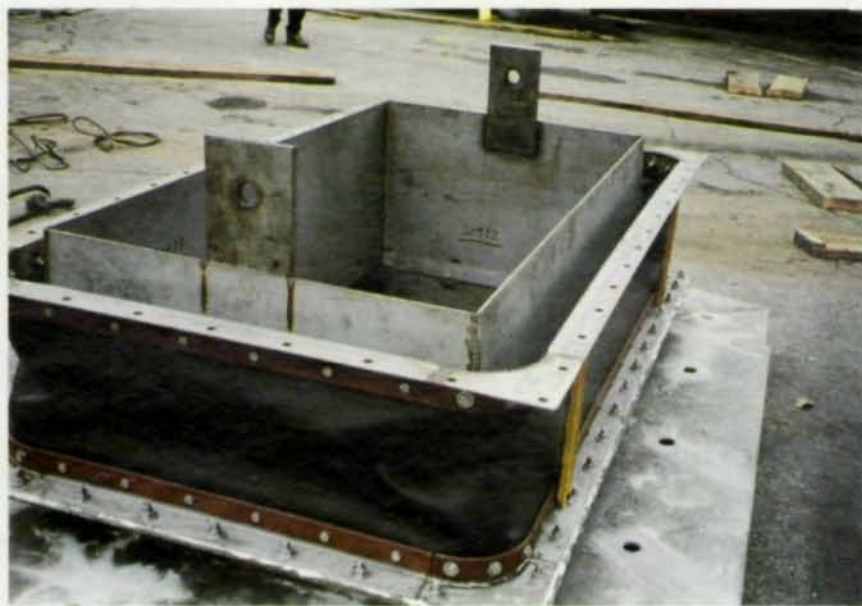
Shown above is the connection assembly that fit on top of the existing stack prior to its installation.
