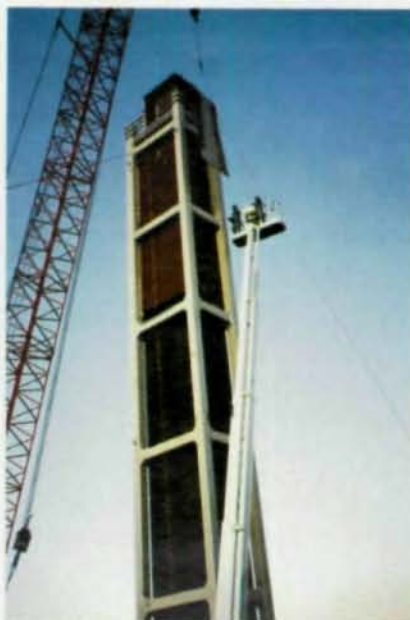
Pictured above is the last plate being fitted into the stack addition.
