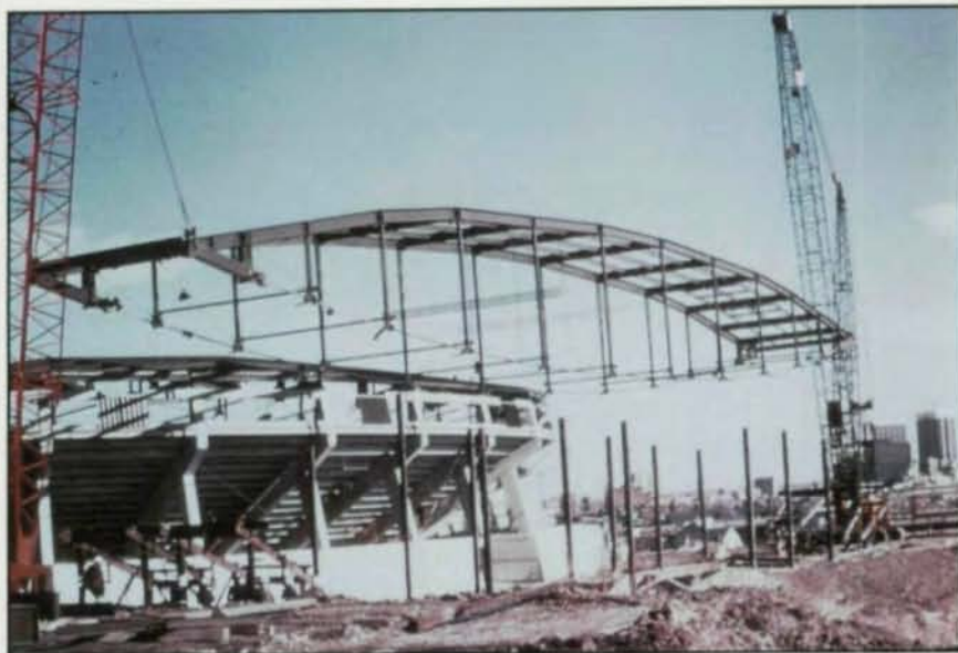
Figure 5: McNichols Sports Arena. Originally designed as a two-way system with cable bottom chords, the system was revised to accommodate redistribution of dead loads from the one-way erection scheme shown above. Cables were added in the opposite direction after erection of all trusses.
