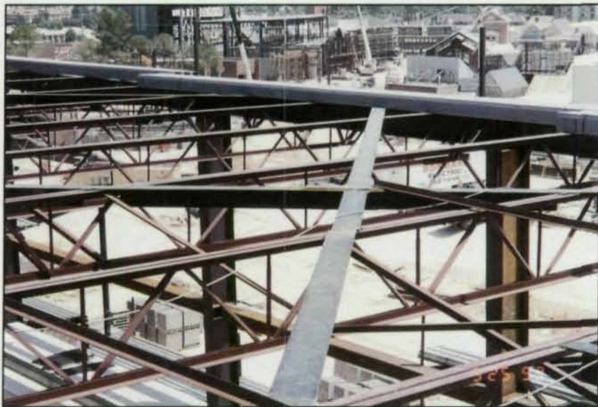
Figure 8: MGM Special Events Center roof structure. WT Shapes notched at each joist were used to brace trusses and carry lateral forces. In this manner, bracing is installed over two or more spans with a single lift of the crane.
