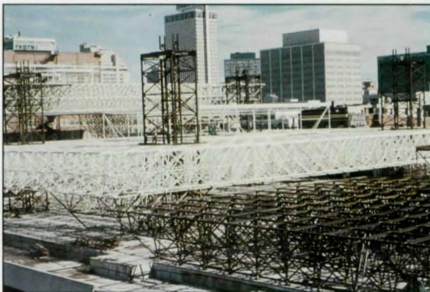
Figure 3 (top): AlamoDome. The primary trusses were designed to be constructed on falsework and lifted by a single crane at each end.
