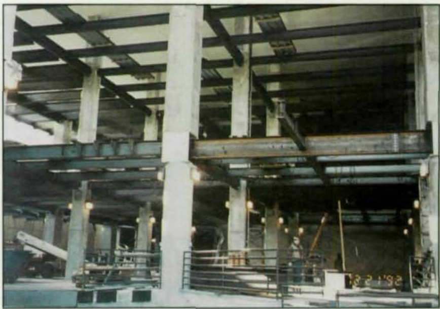
The second and third floor framing was erected to existing columns that supported the fourth floor. Erection was planned to allow the first floor loading dock to maintain its operation.
