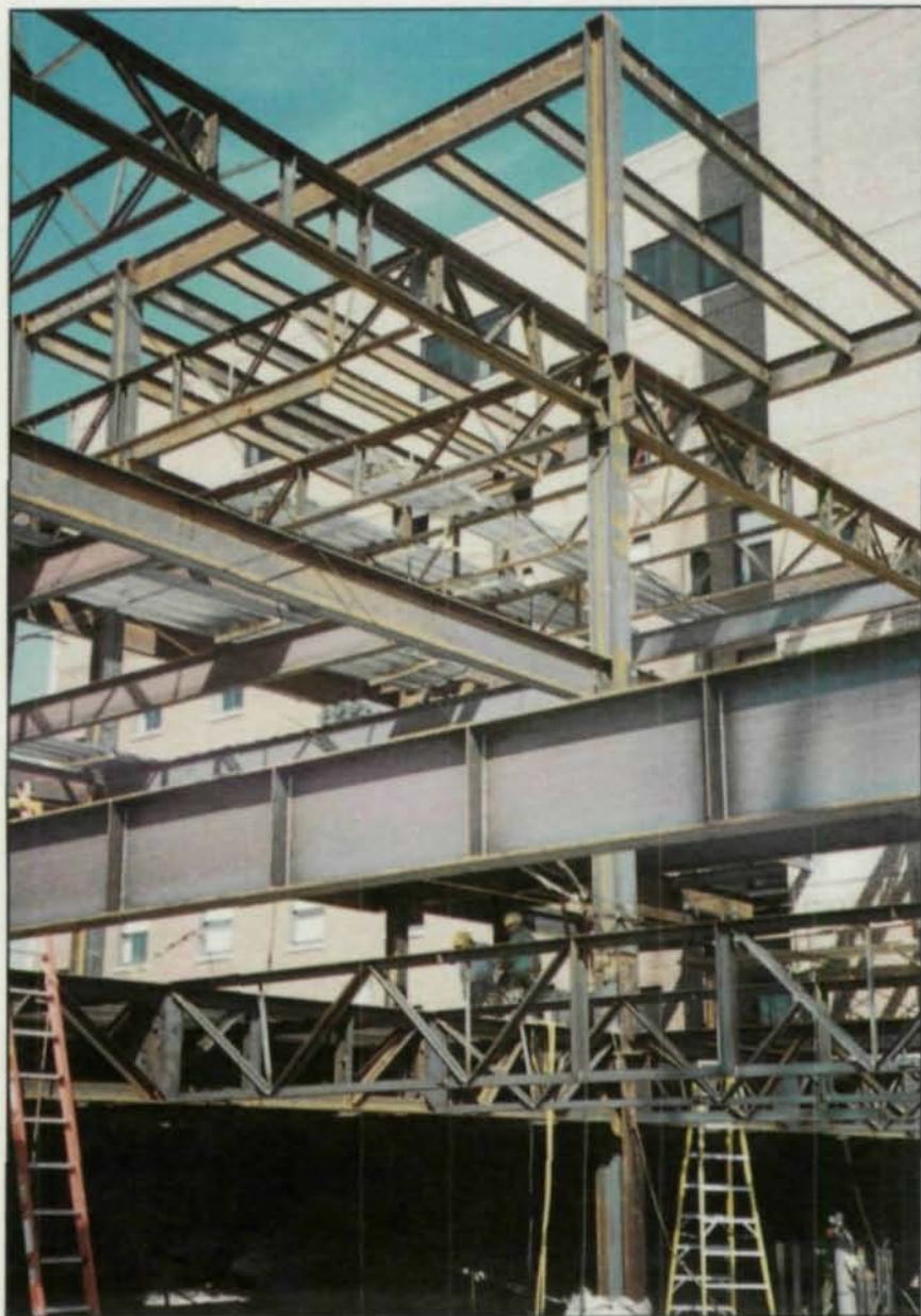
The vertical addition at Columbia Hospital in Milwaukee included three stories plus a penthouse. Vierendeel trusses were used at the first and third levels of the addition.
