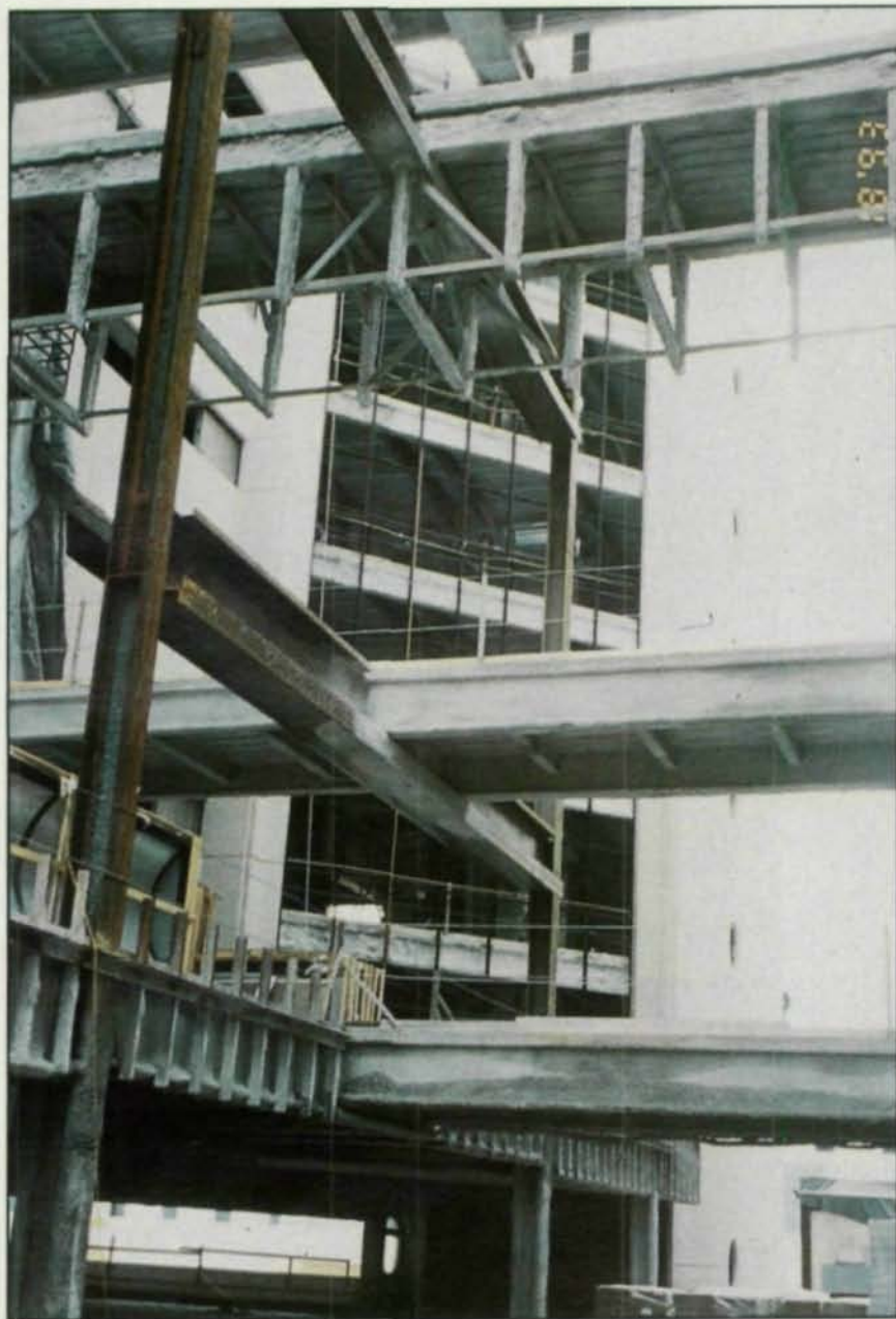
A connector link was constructed to allow passage between the main building and the new east tower. Pictured opposite is one of the three existing footings which was enlarged in order to support a new connector link between the main building and the east tower.
