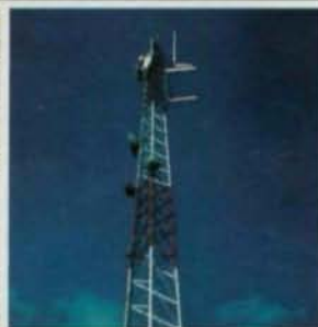
Transmission Towers assembled with UNR-Leavitt HI-Y 50 structural pipe.
