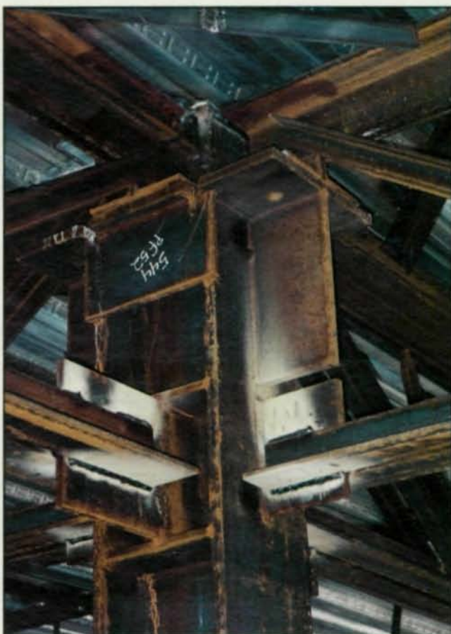
The detail at right shows the vertical reaction and moment connection between orthogonal framing Vierendeel joist girders and a supporting column.
