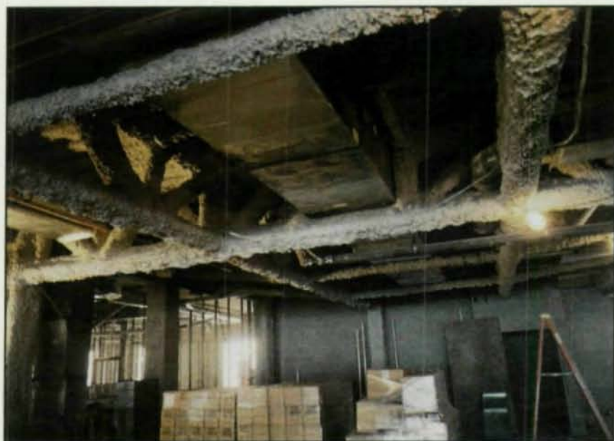
The photo above shows ductwork passing through the Vierendeel panel opening in a typical joist girder, as well as smaller ductwork passing through a variety of additional panel openings.
