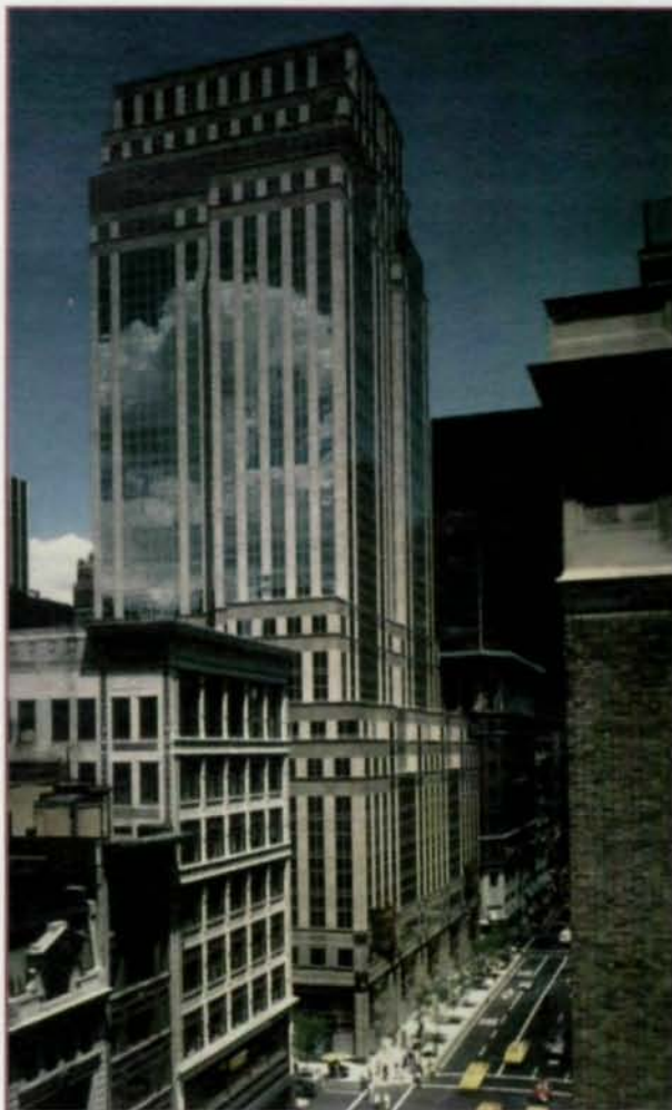
420 Fifth Ave. (left), a 30-story steel-framed office building designed in 1988, was one of the first buildings in New York City to utilize LRFD.
