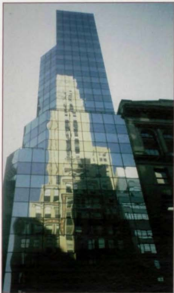
Utilizing LRFD for 546 Fifth Ave. in New York City resulted in a reduction of approximately 15% of total steel tonnage for the building's columns.
