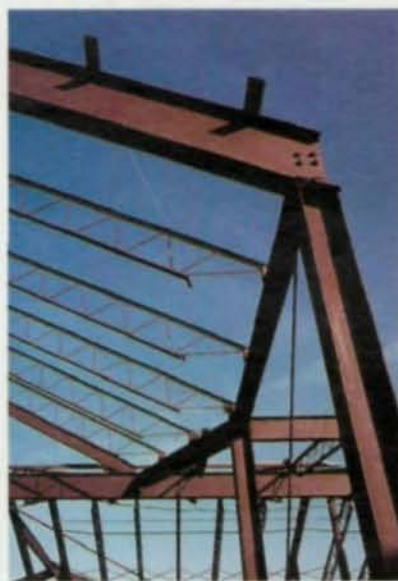
Sloped seat joists can be designed to fit almost any degree of pitch.
