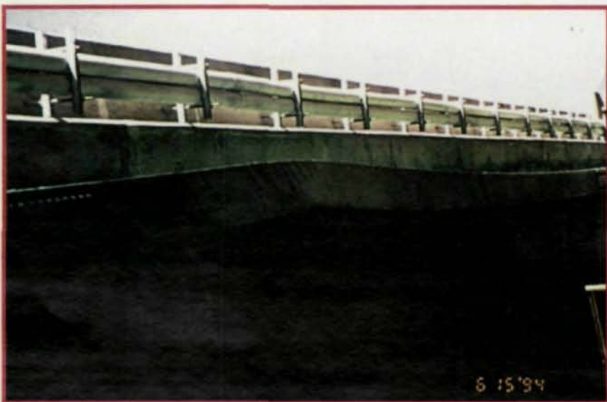
Figure 4 (opposite page): Fractured lower flange of a composite steel girder resulting from over-jacking during heat straightening.
