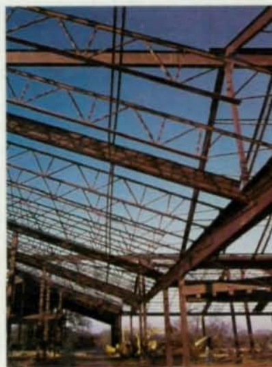
Sloped seat joists work in even the most complex customized framing jobs.
