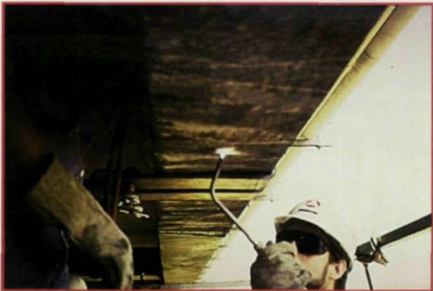
Figure 1: Vee heat in progress at the Mississippi River bridge near Greenville, MS.
