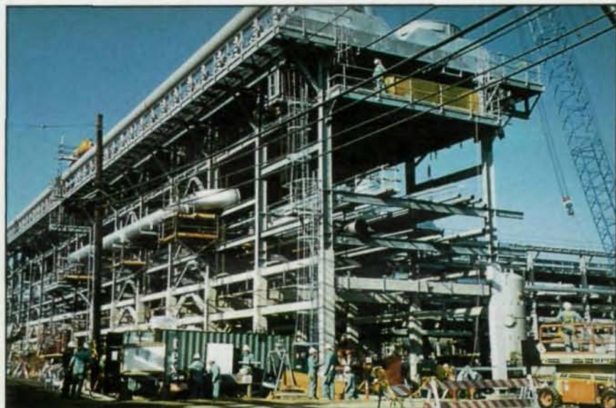
A typical pipeway
