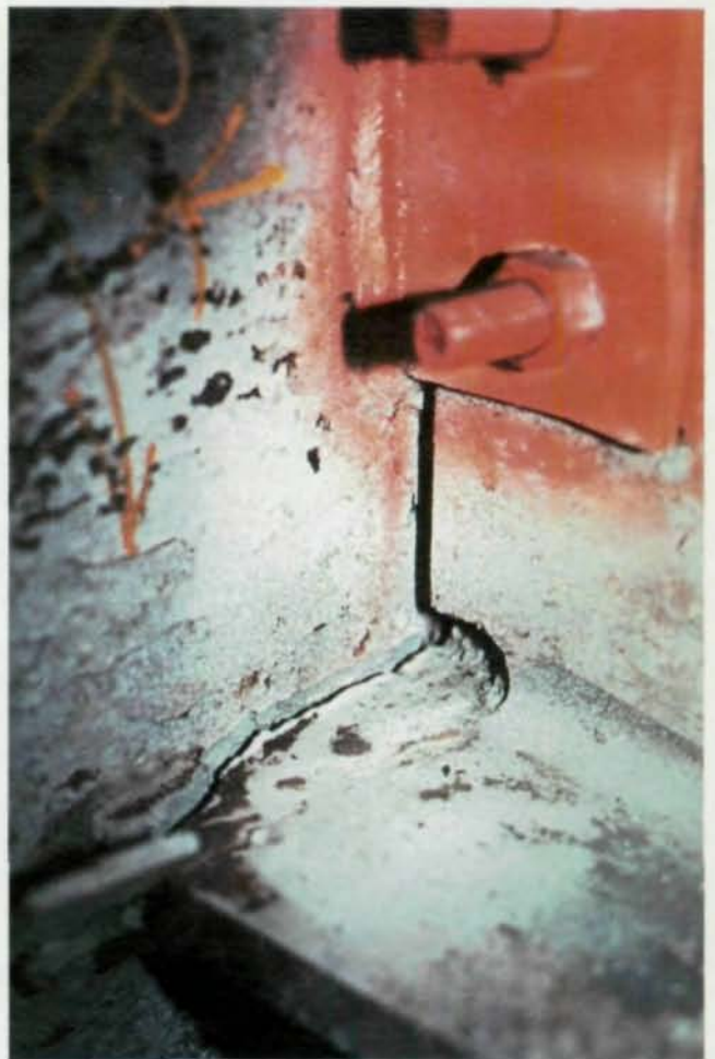
Shown above is a fracture in the heat-affected zone at the weld-column face.
