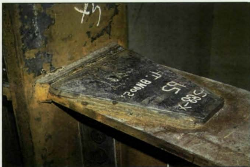
Example of cover plate reinforcement
