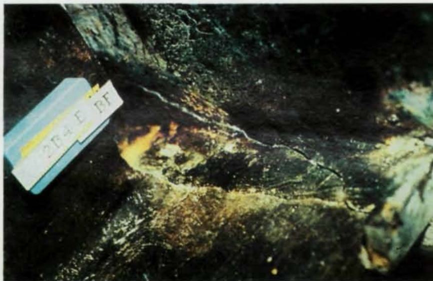
Shown above is an example of weld and column flange fracture. The crack starts in the weld (lower right) and pulls out a divot from the column flange. Photo courtesy of David L. Norris, Western Inspection & Testing.
