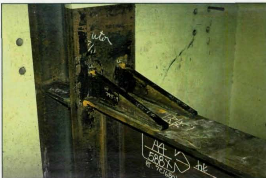
Example of rib reinforcement
