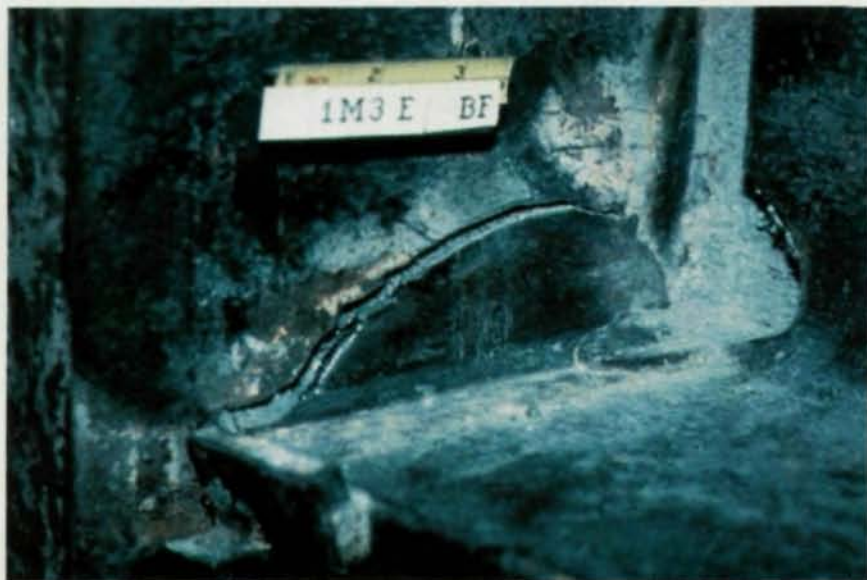
Shown above is another example of lamellar flange tearing (note use of end dam on weld, which is not supposed to be used). Photo courtesy of David L. Norris, Western Inspection & Testing.
