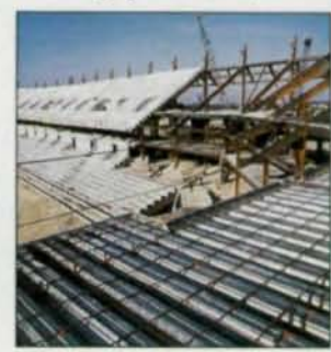
Installing composite deck is faster and easier than poured-in-place concrete.
