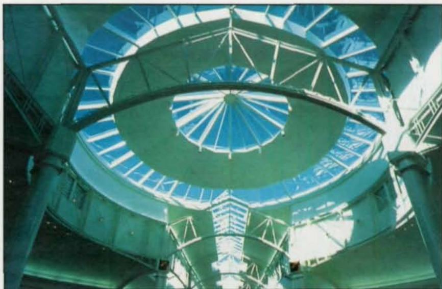
Atop the central court is a huge skylight. The trusses are designed to appear to emanate from the columns and then leap out into the space, where they are linked together by an octagonal-shaped compression ring, from which the second tier of curved linear trusses spring to the top of the space.
