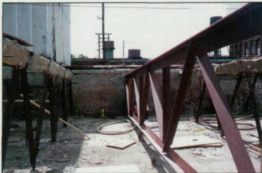
allowed the WT webs to be welded together to form the panel point joints without designing for a large second order moment.
