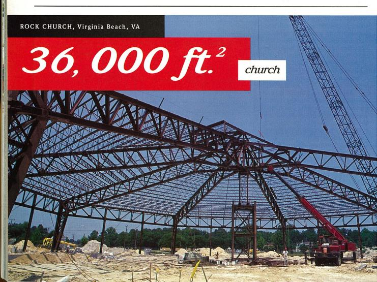
type and number of rows of bridging required depend on the length, spacing and designation of the joists in the area under consideration. The bridging requirements also are affected by wind uplift loading and the type of deck supported by the joists.
