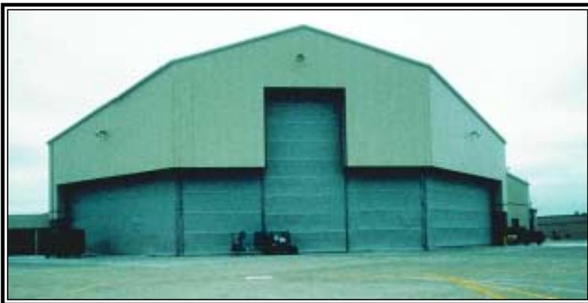
While a square hangar would have been simpler to design, an octagonal building substantially reduced life cycle costs
