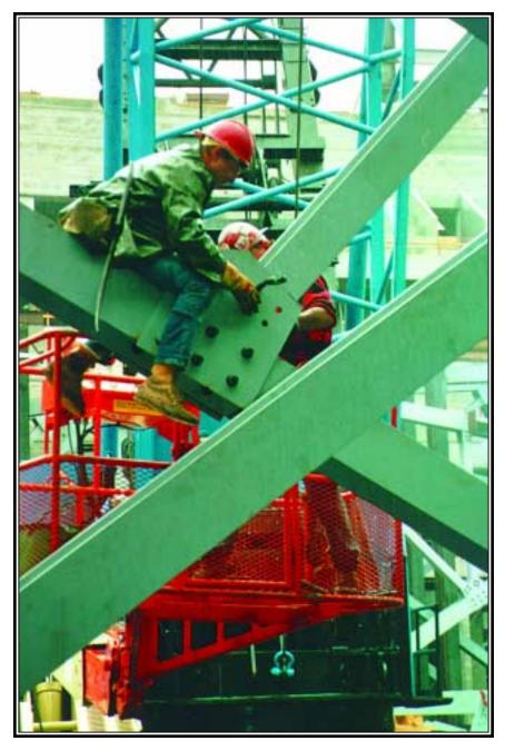
tension members could benefit from the higher grade steel, the top compression chord of the trusses would not see a reduction in weight due to buckling issues. Typically A572 GR-50 steel was used elsewhere. Angles and tubes were 36 ksi and 46 ksi, respectively.
