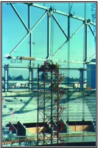
propped cantilever secondary trusses framing into the outboard primary trusses support the 65-ft. roof cantilevers at the north and south ends of the arena. The cantilever areas at the northwest and southeast ends account for almost one quarter of the total roof surface area. Two levels of intermediate beams framing between the primary trusses top and bottom chords are required to carry the various loads associated with a
