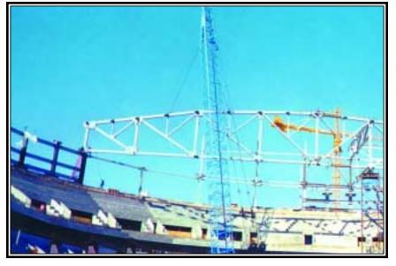
multipurpose arena. The intermediate beams framing into the top chord truss panel points provide bracing for the truss top chord and support the 3-in. 20 gauge acoustical metal roof deck, open web steel joist, and carry a portion of the future suites. The intermediate beams at the bottom chord support an extensive network of catwalks, acoustical clouds, and various rigging loads as well.
