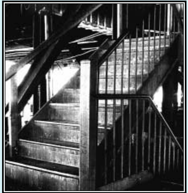
Figure 1: The 850-flight emergency stair system in the World Trade Center performed admirably after the building was bombed in 1993.
