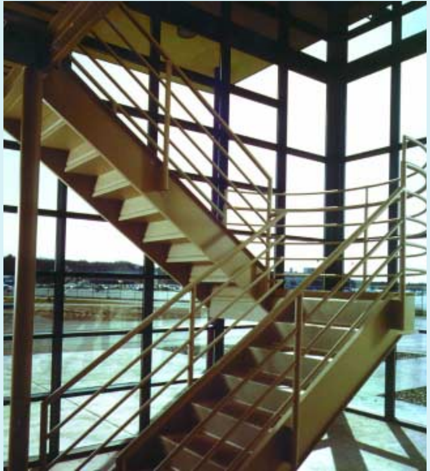
Figure 3: Interconnecting stairs also are highly visible and should be highlighted in drawings and specifications. Photo courtesy of Leers Weinzapfel Associates
