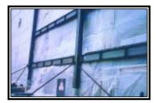
two new stair shafts were required by the owner and the current building codes to extend all the way to ground level. The space available for these new penetrations was very tight and the openings were created by cutting the flange of existing single tees and placing the new structure inside of them. Inches were important and a survey was performed to make sure that the webs of these tees lined up. An analysis of the existing tees revealed that the flanges could be cut and the surfaces epoxied.
