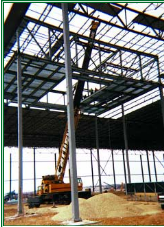
Pictured at left is the penthouse truss framing.
