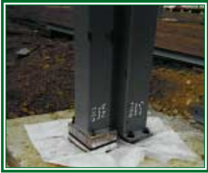
Shown above is the wood isolation base at the column base.
