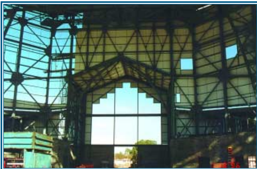
A view from the outside (top) and inside (above) of the nose pocket of the new hangar.
