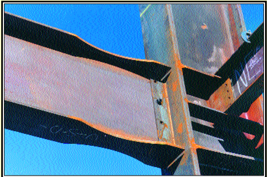
Figures 8a & 8b: Moment frame during erection
