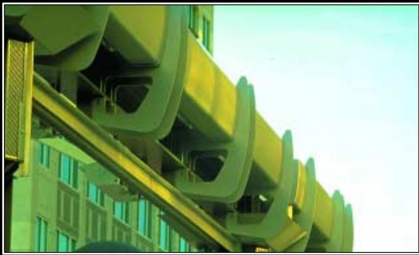
*The columns support W12x58 girders, upon which continuous gutters are mounted, supported by metal "skate blades."*
