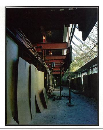
braces. To distribute the upward and downward forces due to seismic overturning, we spread the braces over the maximum number of columns. However, in some areas we removed the concrete fill over the parking garage to ensure that the foundation would not be overstressed.
