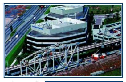
gets truss а longer, the effectiveness of this method is reduced. 300'-long The truss on this project required the introduction of actual expansion joints within the floor system. Using elastomeric bearings pads with angle connections and slotted holes, these expansion joints were added at the approximately third points along the truss. These joints effectively eliminated main member loads from the floor system and any associated steel over-
