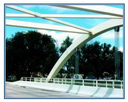
HE NEW REDFIELD RAINBOW ARCH BRIDGE in Redfield, SD, replaced a 1917 two-ribbed reinforced concrete through arch bridge that, while eligible for the National Register of Historic Places, was not economically feasible to rehabilitate.
