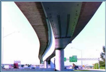
cross-beams attached to diaphragms were provided to transfer the torsional moments to the abutments. Crossbeams also served to anchor negative vertical reactions.
